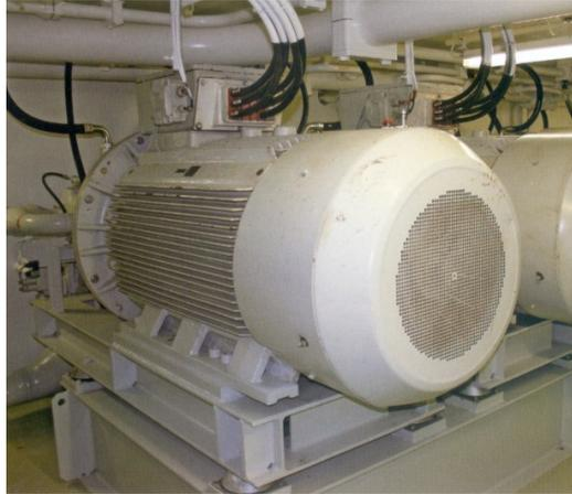
Figure 2.1: asynchronous motor
