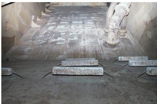
Figure 3.28: Sacrificial anodes in a ballast tank.
