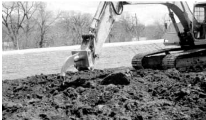
Scarifying the soil during construction significantly improves the chances of any vegetation establishment.
