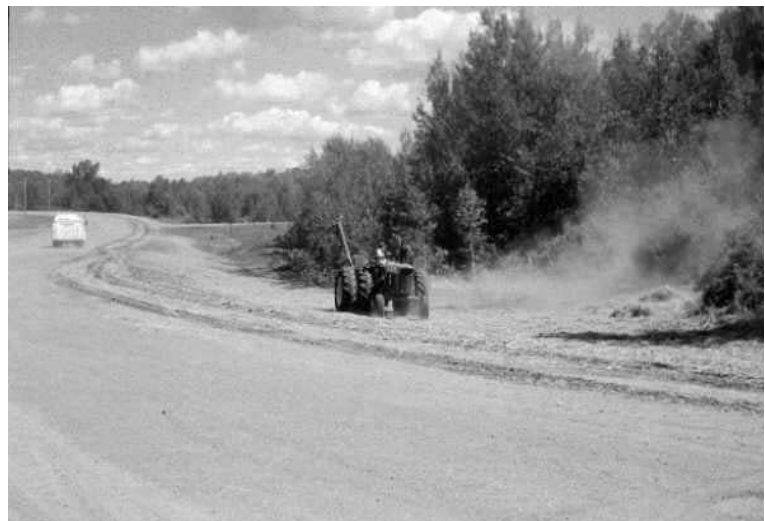
Mulch protects seed and soil from erosion until vegetation can be established.
