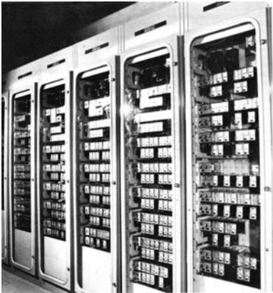
FIGURE 4.24 Cabinets with auxiliary electromagnetic relays, produced by ABB, installed in one of the industrial enterprises.
