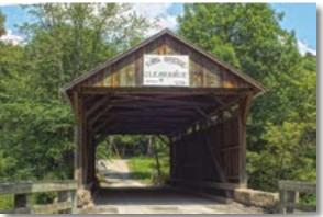
Year Built: 1890 Stream: Hoover Run Length: 46 ft. 6 in. Truss Type: Queenpost Year Listed: 1979 Builder: Unknown Width: 15 ft. 4 in.
