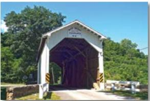
Year Built:1919 Stream: Whiteley Creek Length: 66 ft. 6 in. Truss Type: Queenpost
