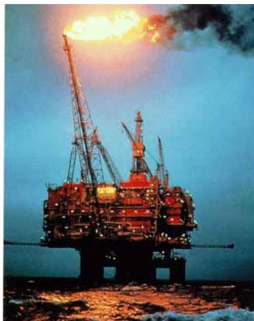
Stronger environmental focus has eliminated continuous flaring and the pilot in many areas. Vapors and flare gas are normally recovered, and only in exceptional situations does flaring occur. To avoid the pilot flame, an ignition
