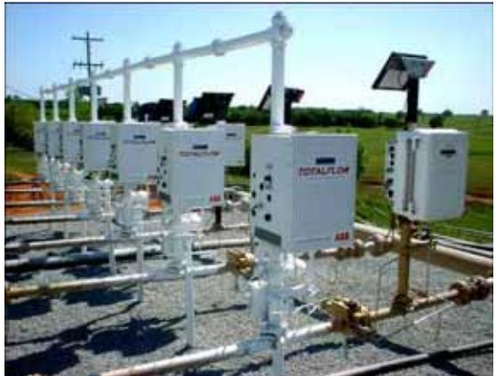
For gas gathering systems, it is common to meter the individual gathering lines into the manifold as shown in this picture. For multiphase flows (combination of gas, oil and water), the high cost of multiphase flow meters often leads to the use of software flow rate estimators that use well test data to calculate actual flow.
