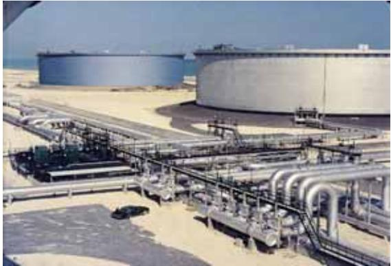
Metering stations allow operators to monitor and manage the natural gas and oil exported from the production installation. These employ specialized meters to measure the natural gas or oil as it flows through the pipeline, without impeding its movement.
