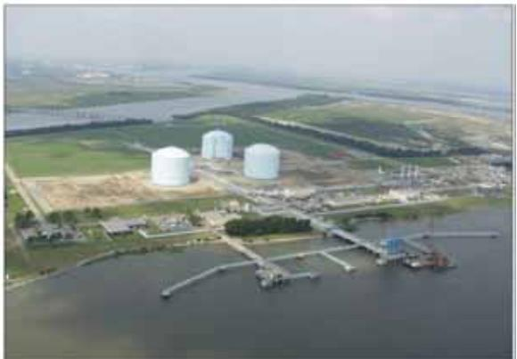
This requires one or more cooling stages. Cooling work consumes 6-10% of the energy to be transported. Special insulated tank LNG carriers are required for transportation, and at the receiving end, a regasification terminal heats the LNG to vaporization for pipeline distribution. *Photo: Cove Point LNG Regas terminal*
