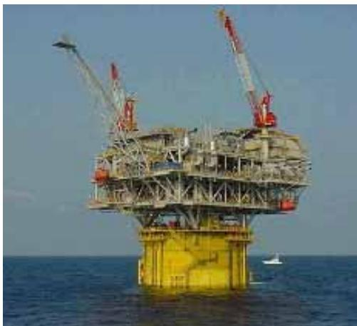
water depths from 300 up to 3,000 meters. SPAR is not an acronym, and is named for its resemblance to a ship's spar. SPARs can support dry completion wells, but are more often used with subsea wells.
