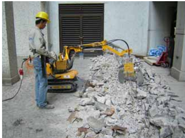
Specially designed crusher for better noise protection
