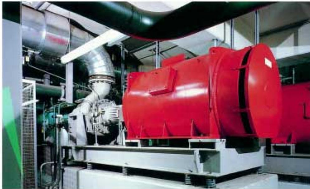
*Speed-controlled three-phase motors for hot-water circulating pump drives for long-distance heating supply*
