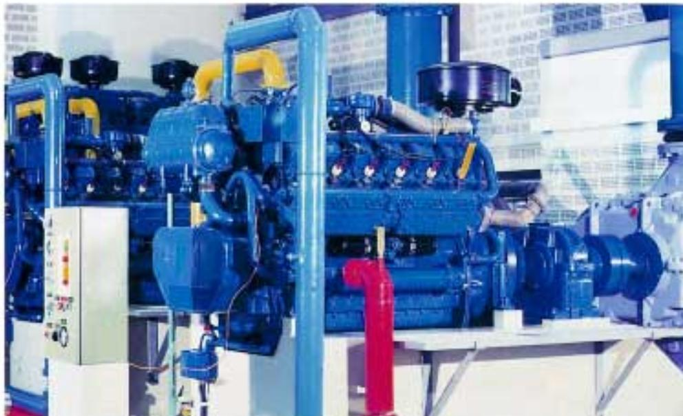
*FLENDER-N-EUPEX coupling and FLENDER-ELPEX coupling in a pump drive*
