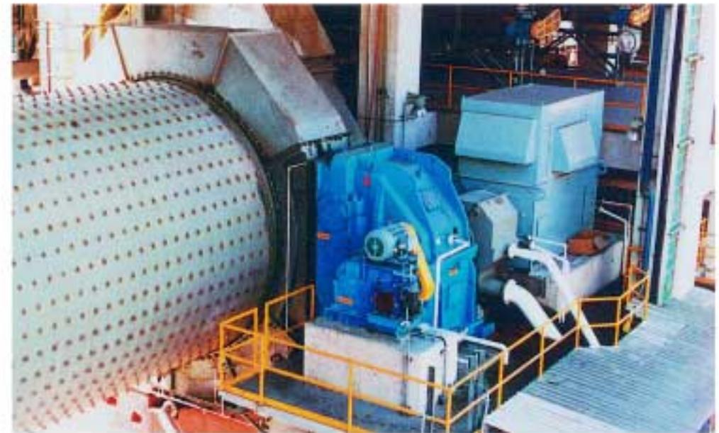
*FLENDER girth gear unit in a tube mill drive*
