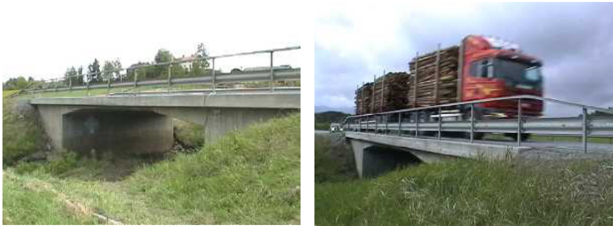
Figure 4.22 Kramfors bridge details: (a) elevation; (b) 7-axle calibration vehicle crossing the bridge.
