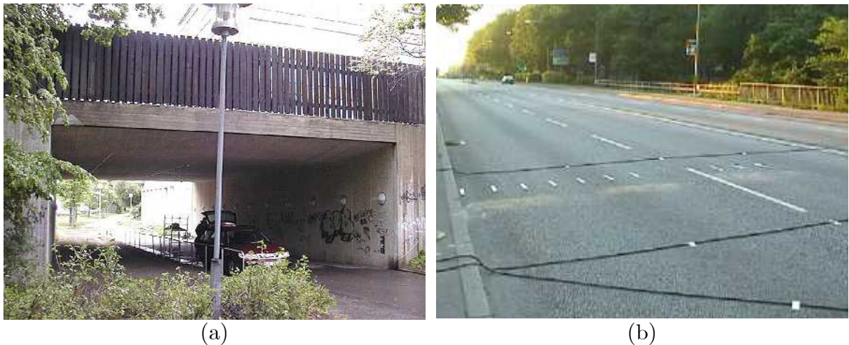
Figure 4.7 Details of Östermalms IP bridge: (a) elevation; (b) layout of pneumatic tubes, reflective strips and sand.
