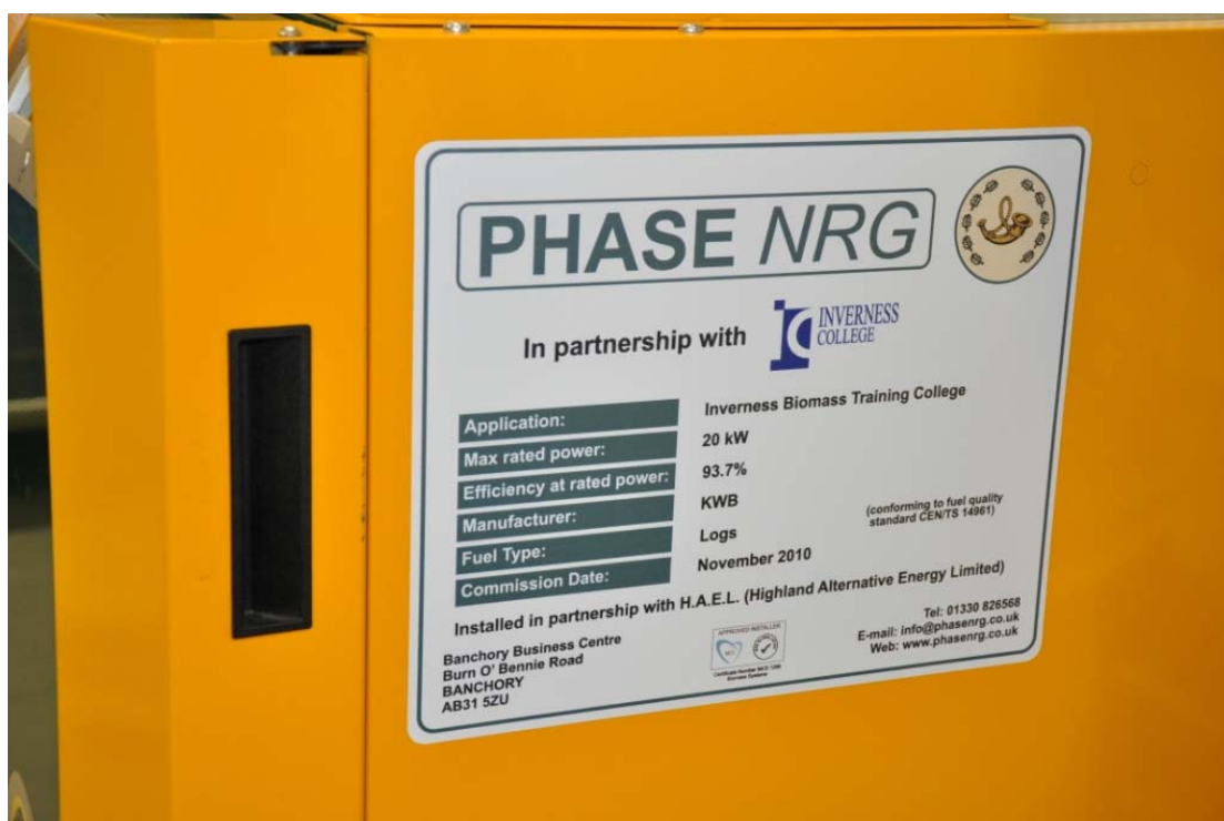
Image 4 Biomass Boiler Display of Technical Information
