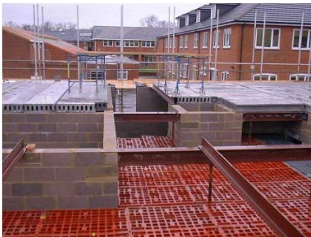
Figure 4-2. Metal decking system. (A) View of a Metal decking system during steel or timber erection work and (B) Metal decking system during masonry work (Source: Health Safety Executive Research Report 302, 2003).
