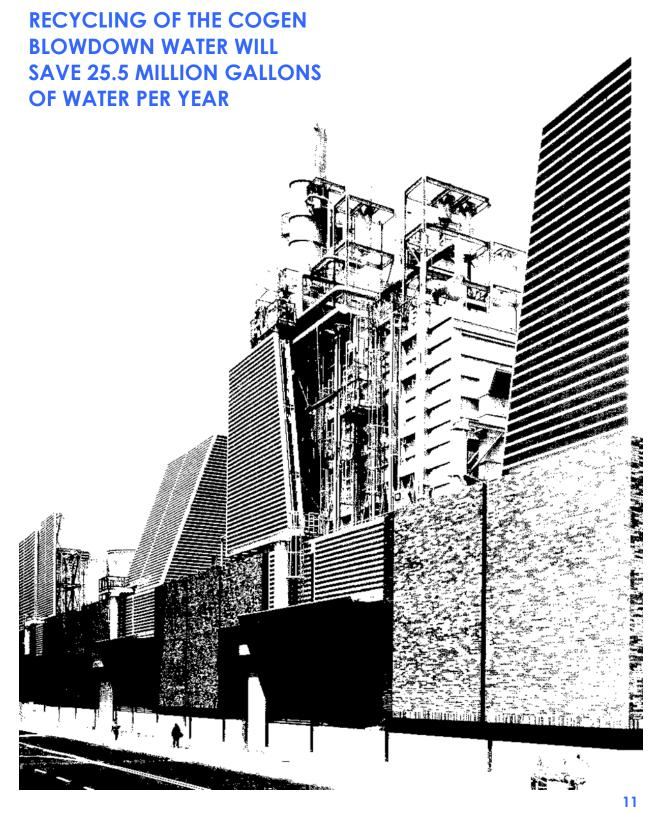
THROUGH INSTALLATION OF AN ACTIVE WATER TREAT-MENT SYSTEM, THE COGEN-ERATION (COGEN) PLANT WILL RECYCLE DAILY BLOW-DOWN WATER AND RETURN IT TO THE COOLING TOWERS
