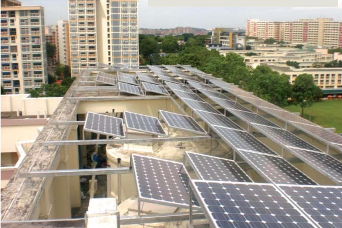
**Figure A.9.1. Typical rooftop PV array layout at Serangoon North Precinct**
