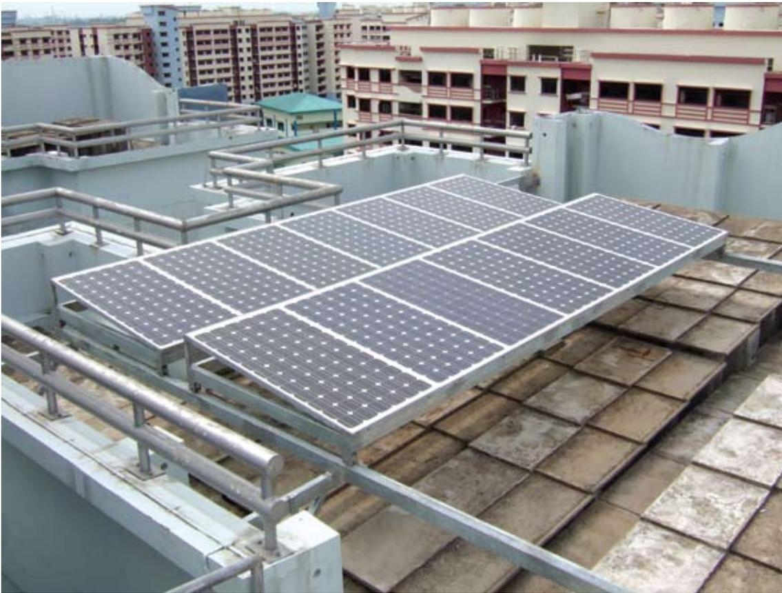
**Figure A.10.1. Typical rooftop PV array layout at Wellington Circle Precinct**
