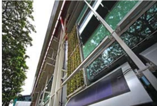
Figure A.1.2. PV array view (PV Sunshade)
