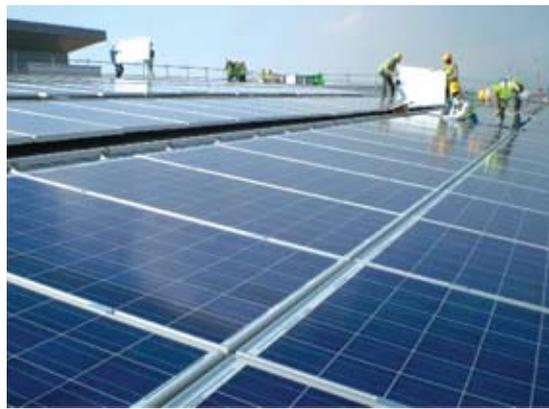
**Figure A.6.3. Installing the REC modules**
