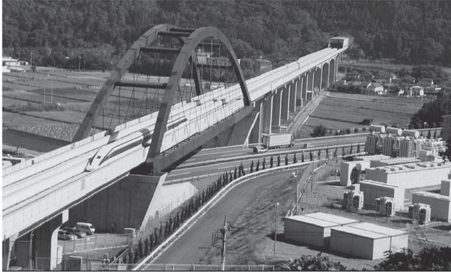
**FIGURE 34.21** YMTL in Yamanashi Prefecture (near Tokyo), Japan. YMTL maglev trains use air-cored LSMs with SC excitation system. (Photo courtesy of Central Japan Railway Company and Railway Technical Research Institute, Tokyo, Japan.)
