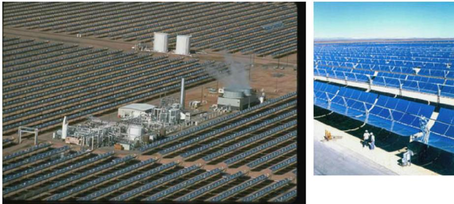
Fig. 4. About 1000 MW of electricity are produced in the California desert at competitive prices by parabolic trough solar concentrators, assisted by fuel, at a capital cost of about \$3000/kW.
