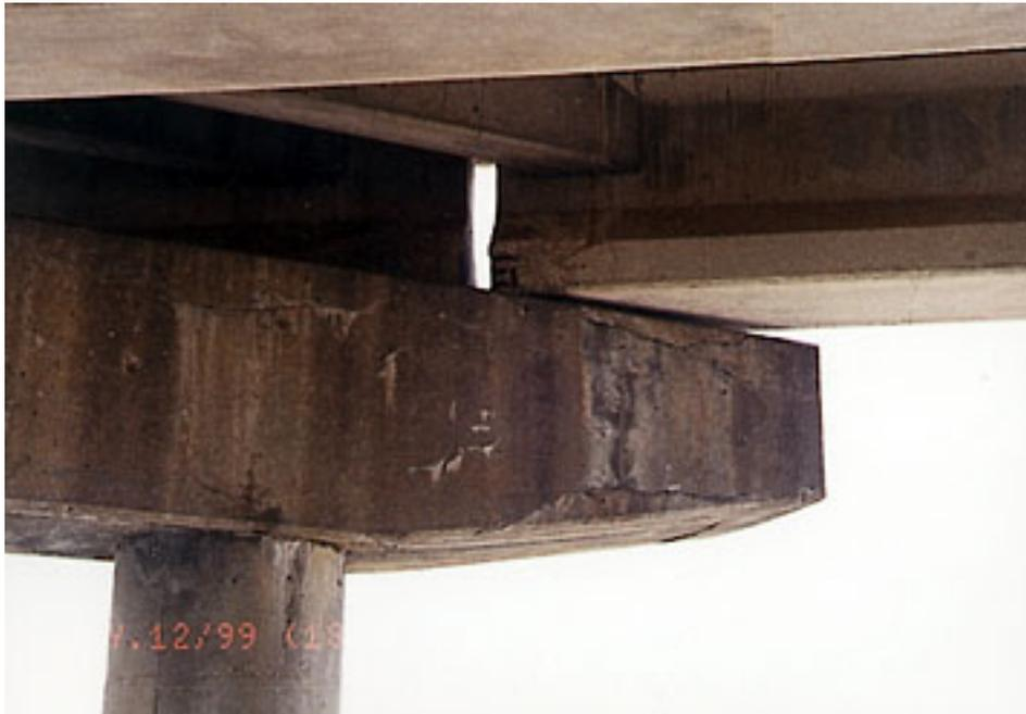
**Figure 2.7 - Severe Deterioration of an Amarillo Bent Cap**
