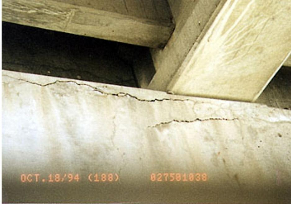
**Figure 2.6 - Top and Side Splitting around Upper Reinforcement in Bent Cap (Amarillo)**
