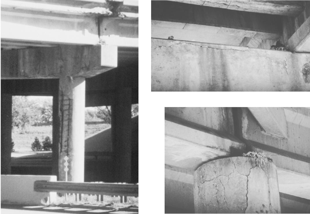
**Figure 5.2 – Severe Substructure Corrosion Damage Due to Defective Expansion Joint**
