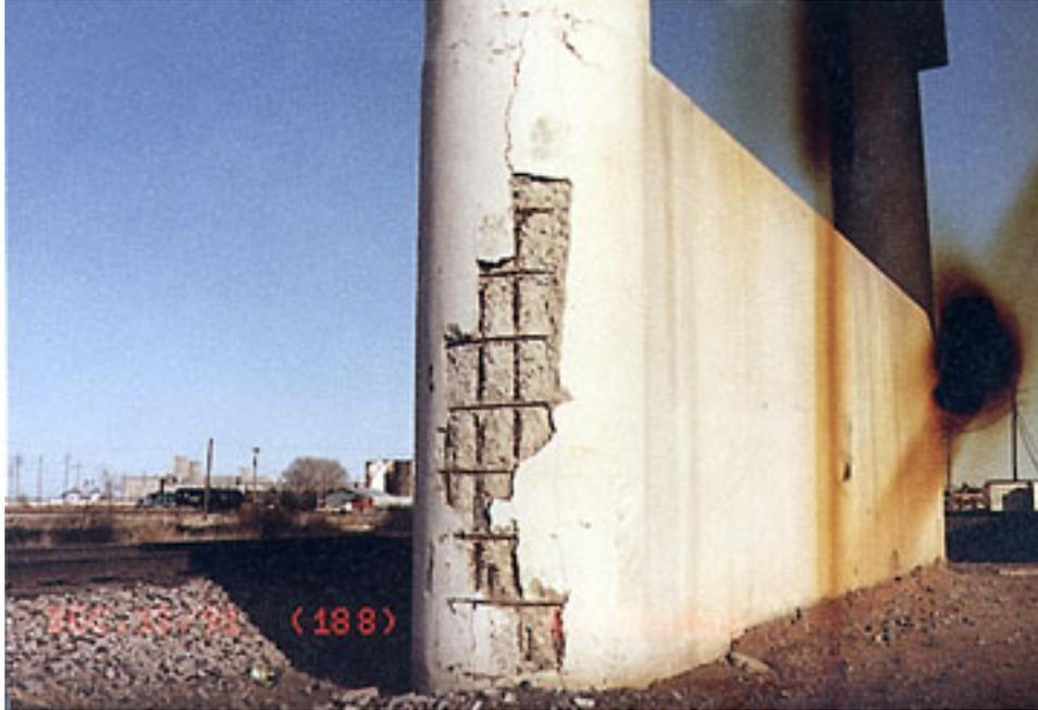
**Figure 2.9 - Deterioration of Columns Due to Salt Laden Snow Piled against the Column**
