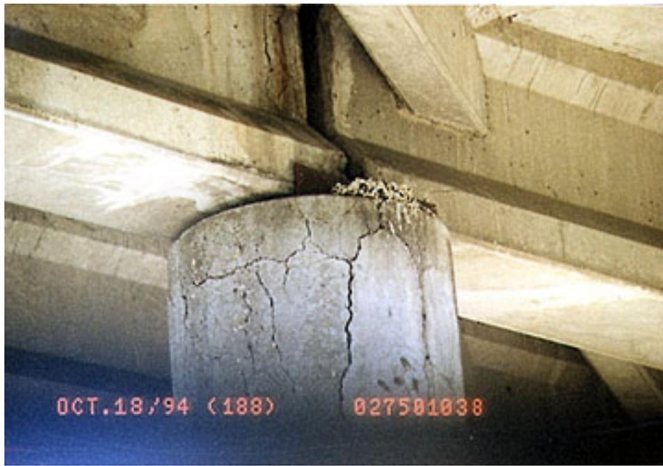
**Figure 2.8 - Single Column Directly under a Construction Joint in Amarillo.**
