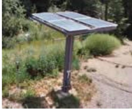
**Tracking solar panel mounts :** Tracking solar panel mounts follow the path of the sun during the day to maximize the solar radiation that the solar panels receive. A single axis tracker tracks the sun east to west and a two-axis tracker tracks the daily east to west movement of the sun and the seasonal declination movement of the sun.
