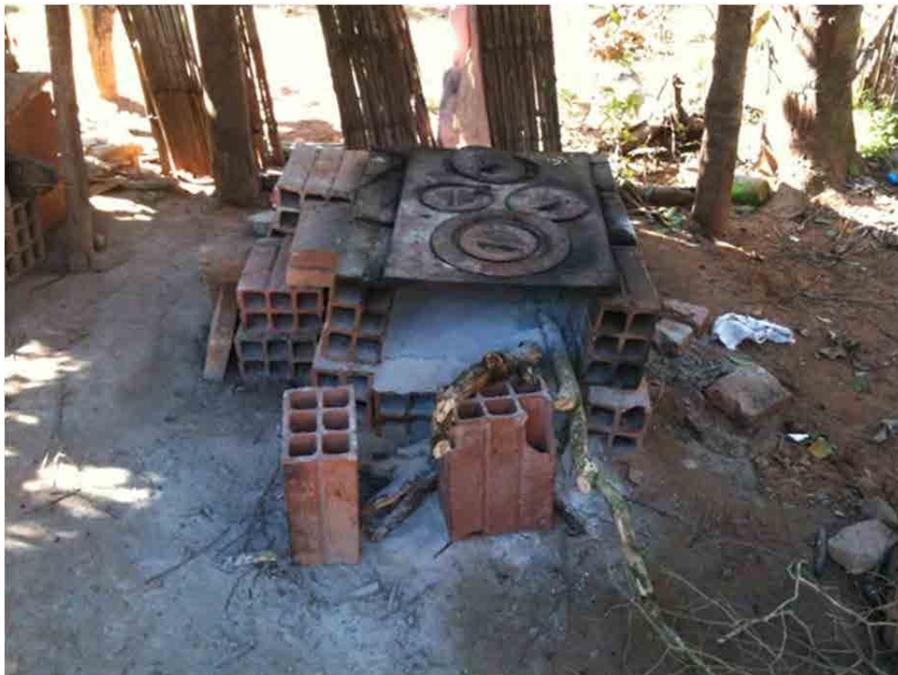
Fig 24. An example of the improper use of fogon materials - the equivalent of open fire cooking.
