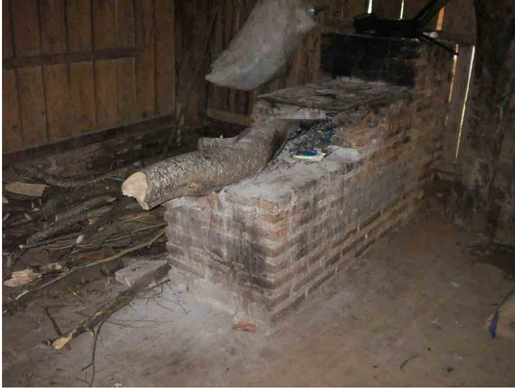
Fig. 17. Fogon with large piece of wood. Note the damage of missing bricks under the plancha .
