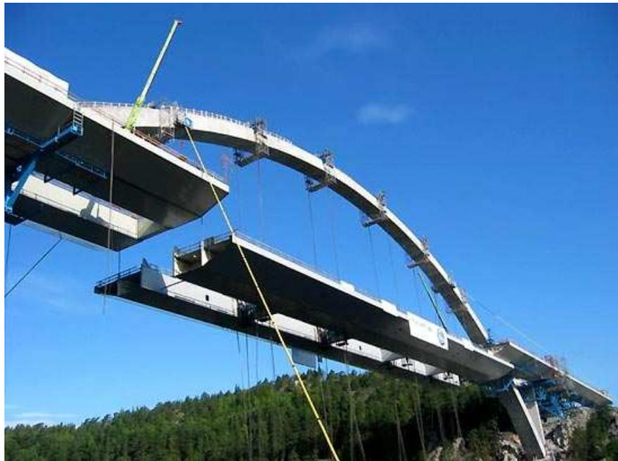
**Figure 1.4** The central section of the bridge is lift in its final position.
