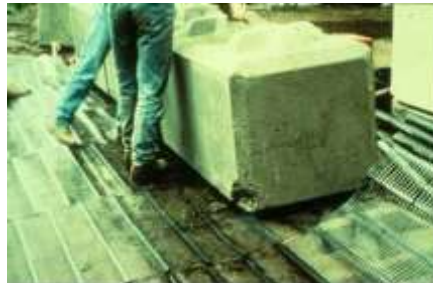
Figure 19: Example of large wet-cast concrete modular block.
