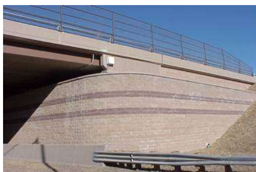
Figure 22: Founders/Meadows GRS bridge abutment.
