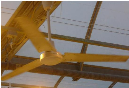
**Figure 14. Paddle fan to increase vertical air movement and therefore evapotranspiration. This is important for the prevention of tipburn.**
