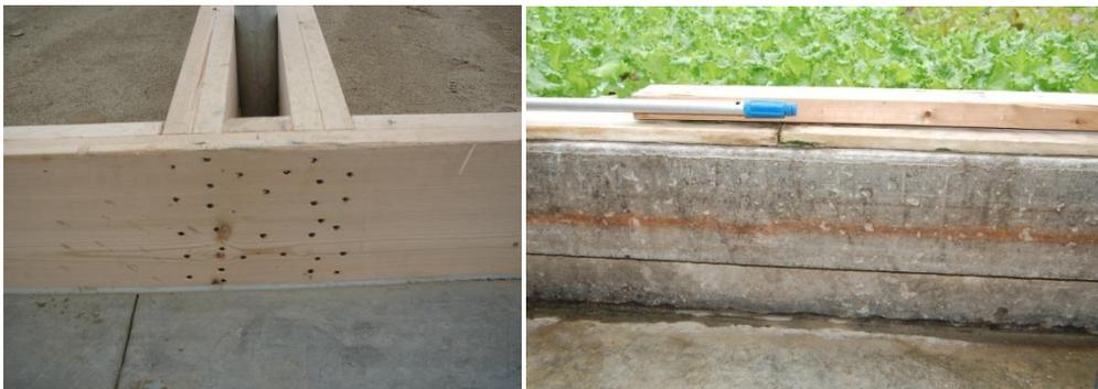
Figure 13. Edge of pond detail. The inside edges of two separate ponds made of wood and separated by structural members is shown on left. The right hand picture shows a concrete pond.
