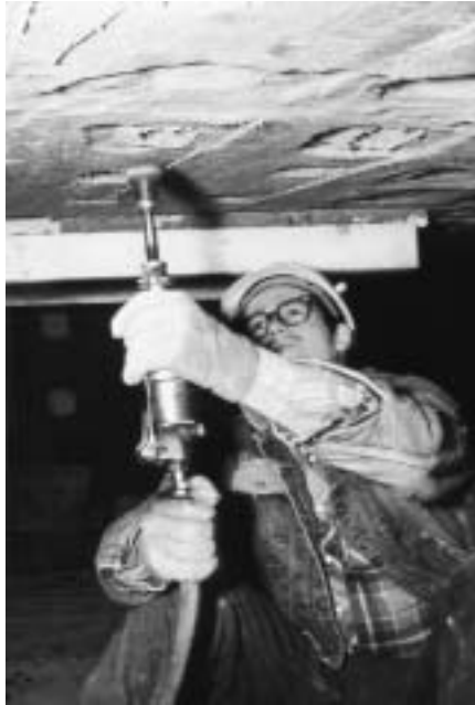
Peening. Plastic adjacent to anchors should be lightly rammed up and around the anchors to give a tighter seal.
