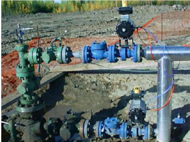
hole with casing, evaluating the pressure and temperature of the formation, and then installing the proper equipment to ensure an efficient flow of natural gas from the well. The well flow is controlled with a choke.
