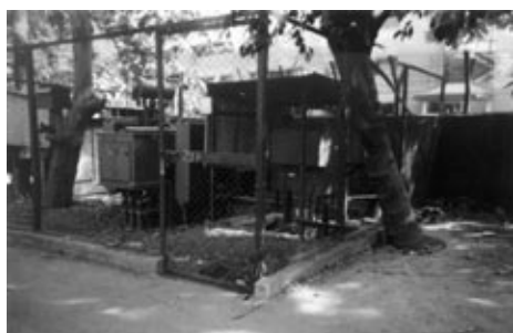
Fig. B39 : Outdoor substations without enclosures
