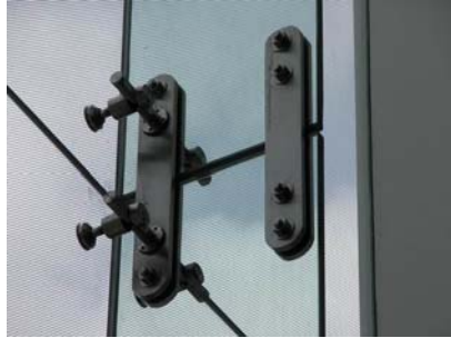
Figure 2.21 Splice plates at the fin sections act to tie point-fixed glass to fins (ASIDI).
