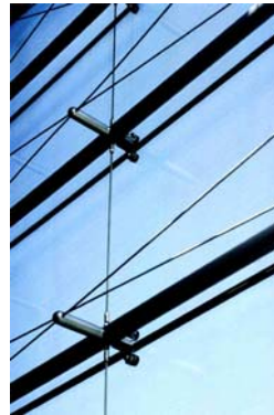
Figure 7.15 Example of horizontal glass grid. Figure 7.16 Mid-span connection of long horizontal IGU.
