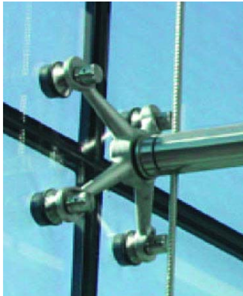
Figure 2.37 Point-fixed insulated glass with butt-glazing (ASIDI).
