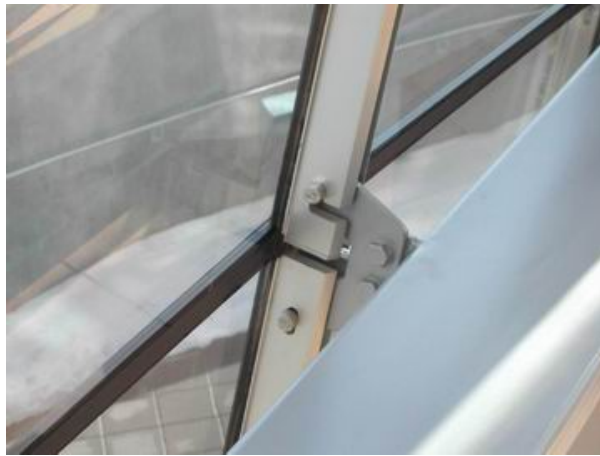
Figure 2.36 Detail of a panelized glazing system (ASIDI).
