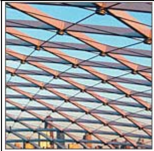
Figure 6.9 An overhead curved gridshell structure (Novum Structures 2008). 10
