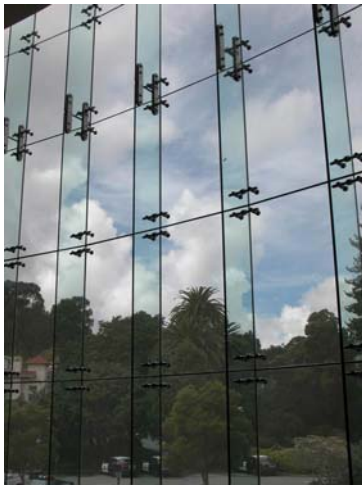
Figure 2.20 Glass fins are set perpendicular to the glass plane to resist lateral loads (ASIDI).
