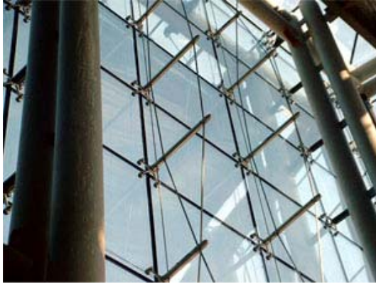
Figure 2.16 Cable trusses span between tubular steel infrastructure (ASIDI).
