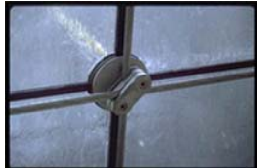
Figure 1.24 UBS Tower cable net facade; water penetration test in progress (ASIDI).
