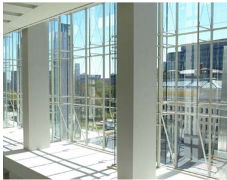
Figure 7.17 Vertically oriented glass grid with truss at each gridline.
