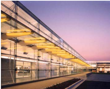
Figure 7.15 Example of horizontal glass grid. Figure 7.16 Mid-span connection of long horizontal IGU.
