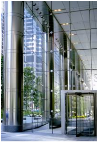
Figure 2.17 UBS Tower, Chicago; flat cable net, Lohan Caprille Goetsch Architects (ASIDI).
