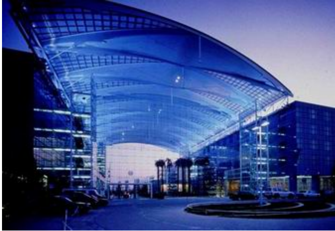
Figure 1.20 Cable net at the Kempinski Hotel, Munich; Murphy/Jahn architect with Schlaich Bergermann engineers (photo courtesy of Schlaich Bergermann).
