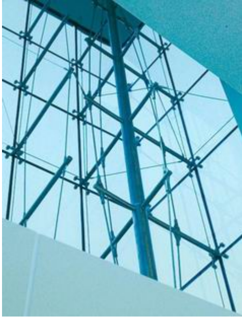
Figure 6.7 A corner truss in a cable truss system.
