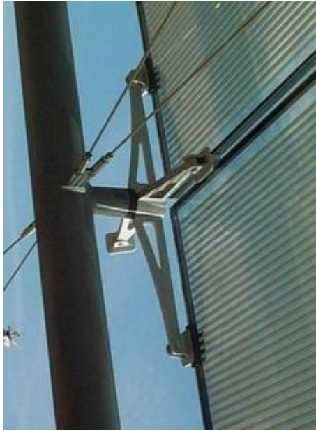
Figure 2.38 Detail of a point-fixed clamped system (ASIDI).
