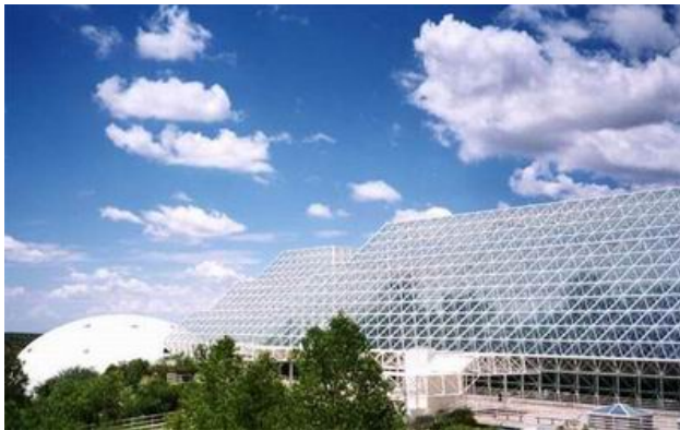
Figure 6.3 Biosphere 2; a large glass-clad space frame enclosure (Biosphere 2 2006).
