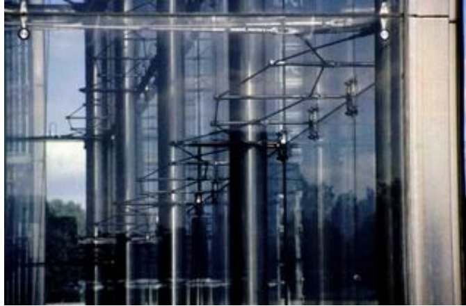
Figure 1.17 Cable trusses of Les Serres, Paris; Adrien Fainsilber with RFR (author's image).
