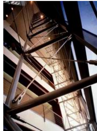
Figure 2.7 Simple truss system with internal tension rod bracing and rectangular exterior chord (ASIDI).
