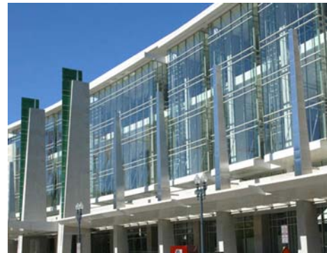
Figure 7.18 Example of vertical glass grid with horizontal module providing visual accent.
