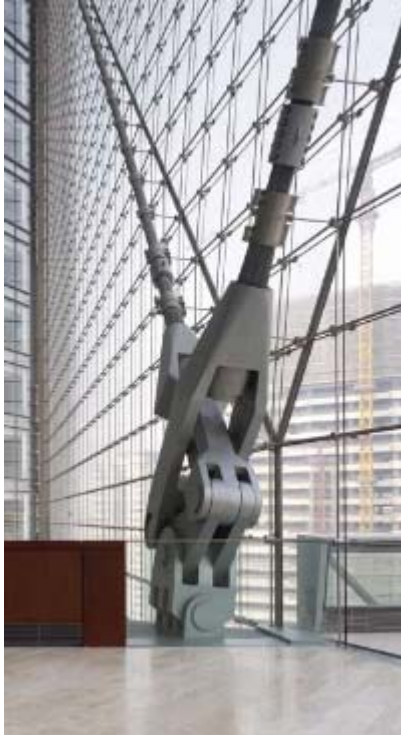
Figure 6.13 Rocker arm detail on New Beijing Poly Plaza cable net; SOM architect, (Griffith 2007b).
