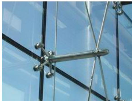
Figure 2.15 The spreader is the only compression element in this cable truss system (ASIDI).
