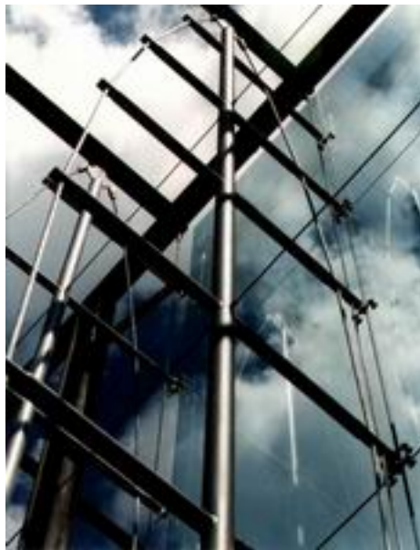
Figure 2.9 A planar mast truss with point-fixed glass during installation (ASIDI).
