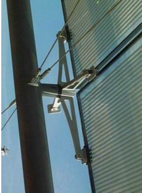
Figure 6.17 Point-fixed clamped system with insulated-laminated glass during installation.
