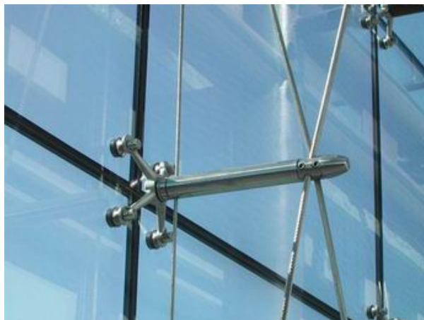
Figure 6.16 Point-fixed bolted system with spider fitting and insulated glass.
