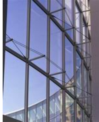
Figure 6.8 Horizontal cable truss bracing a rectangular tube.
