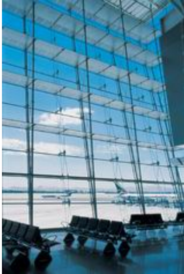
Figure 2.4 Simple trusses alternate with vertical cable trusses (ASIDI).
