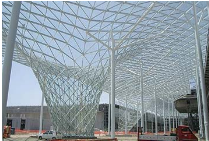
Figure 2.11 Gridshell glass canopy (New Trade Fair in Milan n.d.)
