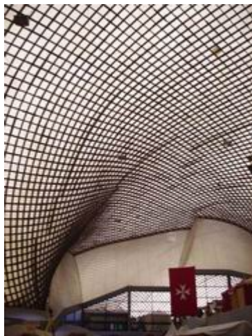
Figure 2.10 Mannheim Multihalle, Germany; grid shell by Frie Otto with Burro Happold, 1975 (Griel 2006)
