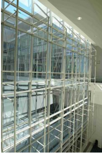
Figure 2.3 Simple trusses set at each vertical grid module (ASIDI).
