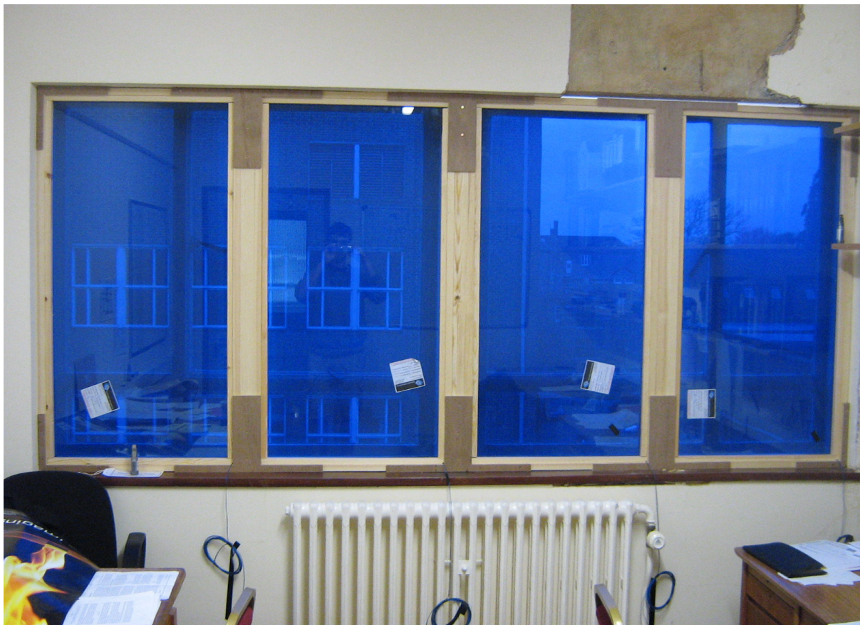
Figure.4c shows all the SPD windows unconnected and switched off. The windows display a blue tint, and the connector wires can be seen hanging from the windows.
