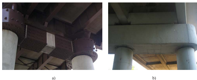
Fig. 14. (a) Bent cap retrofit in Missouri using steel encasement; (b) a bent cap retrofit using reinforced concrete encasement in Tennessee (Dayview Plantation Road over I-40)
