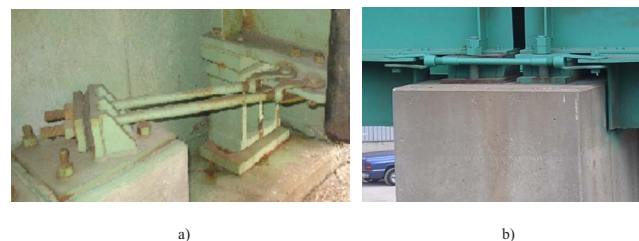
Fig. 10. (a) Restrainer bars in Indiana resisting longitudinal and lateral displacements; (b) restrainer bars in Missouri (Poplar Street Complex) joining adjacent girders at a center span
