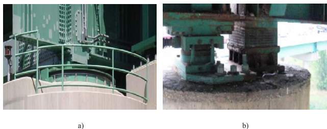
Fig. 6. (a) Friction pendulum (sliding) bearing found on the Hernando DeSoto Bridge in Tennessee; (b) a friction bearing used in conjunction with an elastomeric bearing in Illinois
