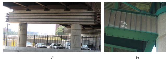
Fig. 13. (a) Bent cap retrofit in Missouri using posttensioned rods; (b) a bent cap retrofit in Illinois using shear reinforcement and confinement on the end regions of the bent cap
