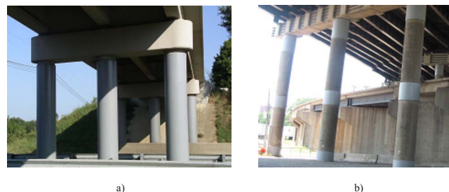
Fig. 16. (a) Full column steel jacketing used in Tennessee (SR 196 over I-40); (b) partial height steel jacketing in Missouri focusing on plastic hinge regions of the columns
