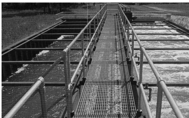
Figure 3.4 Sequencing Batch Reactor (SBR)
