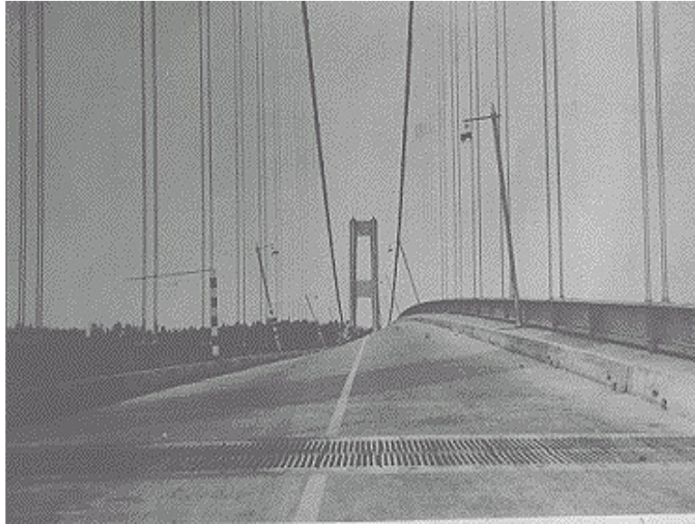
Figure 11.1: This image shows some of the kind of vibration experienced by the Tacoma Narrows Bridge due to aeroelastic flutter.
