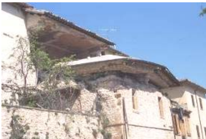
Figure 1.1 Example of a) Out-of-plane collapse of a wall with R.C. tie beams, b) roof hammering the masonry walls, (Binda 2006a).
