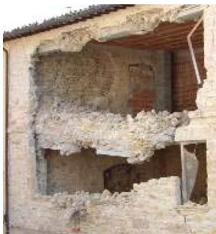
Figure 1.1 Example of a) Out-of-plane collapse of a wall with R.C. tie beams, b) roof hammering the masonry walls, (Binda 2006a).
