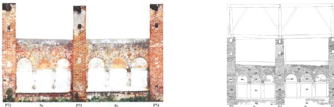
Figure 3.14 Rectified picture and detailed restitution of the damaged wall of a stable in a rural building in Milan. Source POLIMI.
