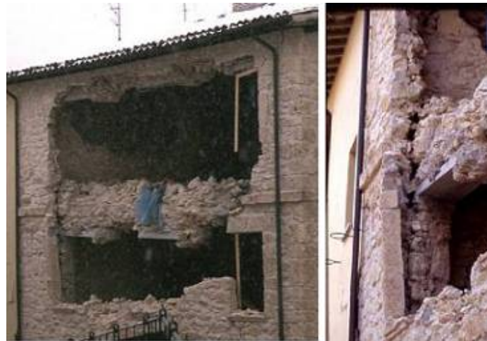
Figure 5.26 Separation of masonry leaves and collapse under out-of-plane actions, (Binda 2006a, b).
