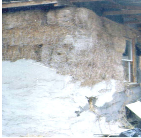
Figure 29. Northwest wall section of House No.2 - remains unfinished for 3yrs now.
