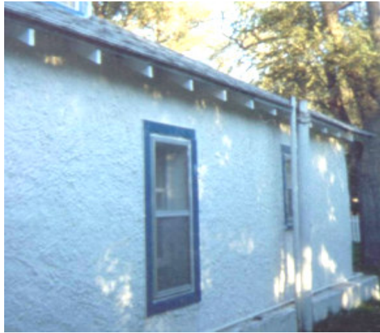
Figure17. An early 19 th century straw-bale home uses lime in its plaster.
