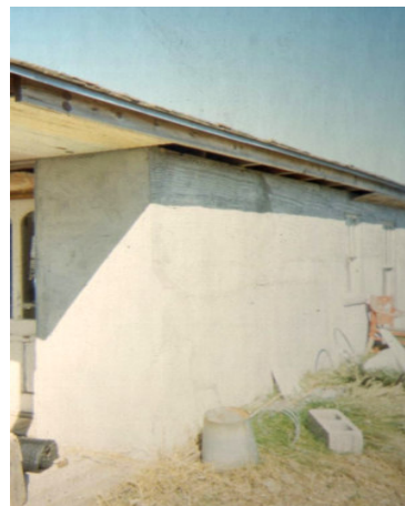
Figure 26. House No.3 western wall with more appropriate overhang length
