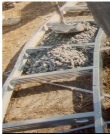
Figure 20. A simplified example of an infill gravel foundation system
