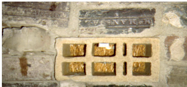
Figure 15. A straw-bale “truth window”
