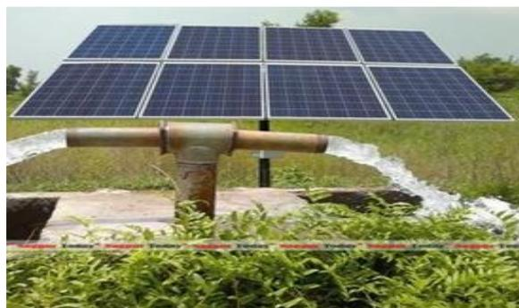
which can easily be borne by the Gram Panchayat. The unit runs on solar power of 1800 Watt panels and produces 10000 Litres of purified water every day.
