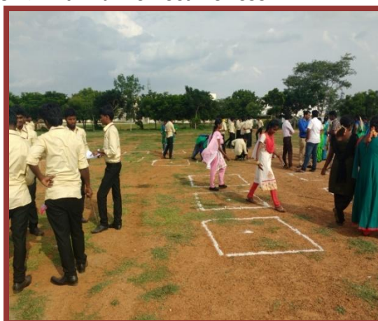
Students are in progress about foundation marking in Field Workshop
