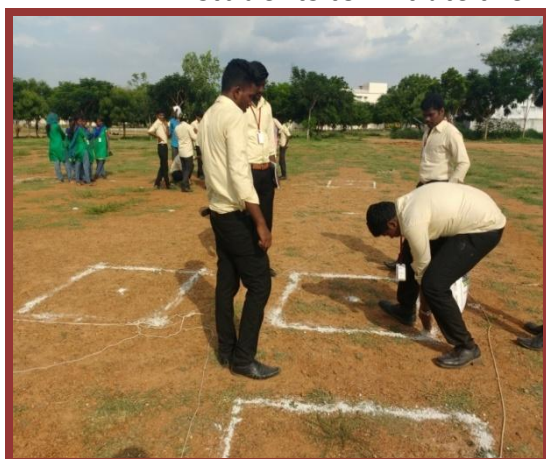
Students are in progress about foundation marking in Field Workshop
