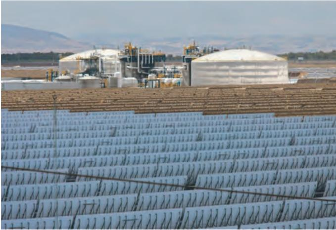
**Figure 11.56** | Two-tank molten-salt indirect storage system at the 50 MW Andasol 1 parabolic trough plant in Spain. Source: Photo courtesy of Solar Millennium.
