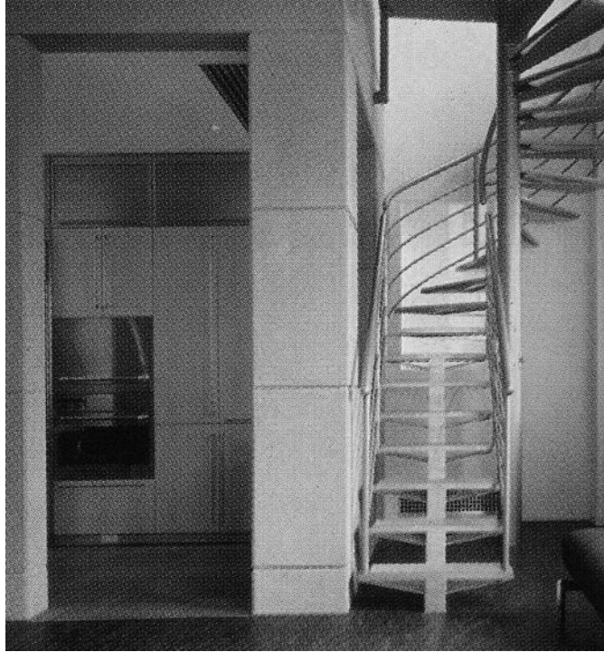
Figure 6. A narrow stairway with variation in tread size (Photographer: Michael Moran Photography).
