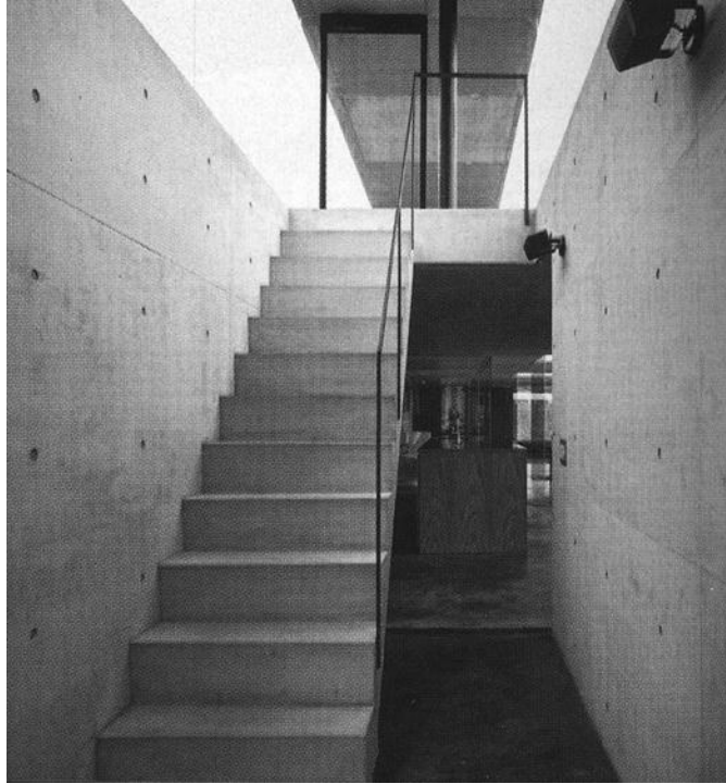
Figure 4. A stairway with a thin truncated handrail, inadequate balustrades, and low visual contrast on the tread edges (Photographer: Toshiyuki Yano).
