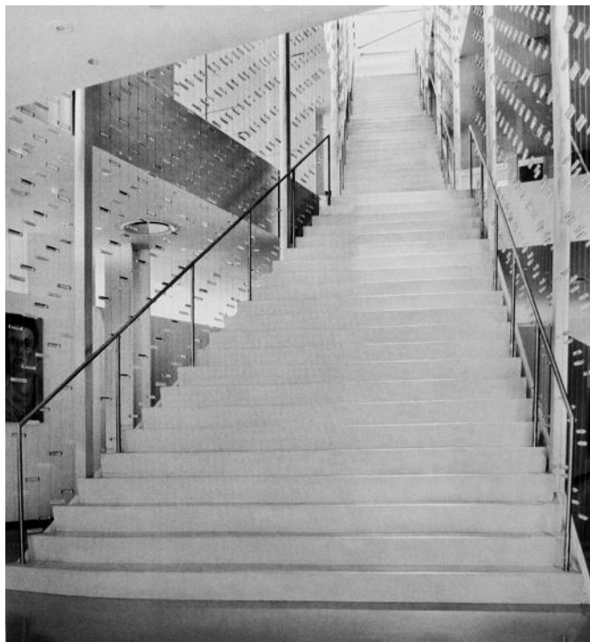
Figure 7. A stairway with an excessive stair run length (Photographer: Elizabeth Felicella).
