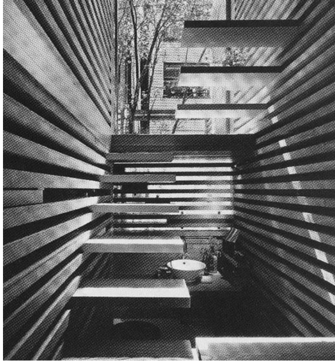
Figure 5. Visual distractions in an open riser stairway (Photographer: Kouji Okamoto / Techni Staff).
