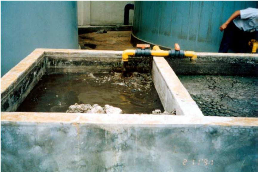
Fig. 6.5.1. A pair of sludge drying beds with one (RHS) in drying phase while the other (LHS) is in filling phase. Splash plates need to be placed under the feed pipes to reduce disruption of the sand layer beneath.
