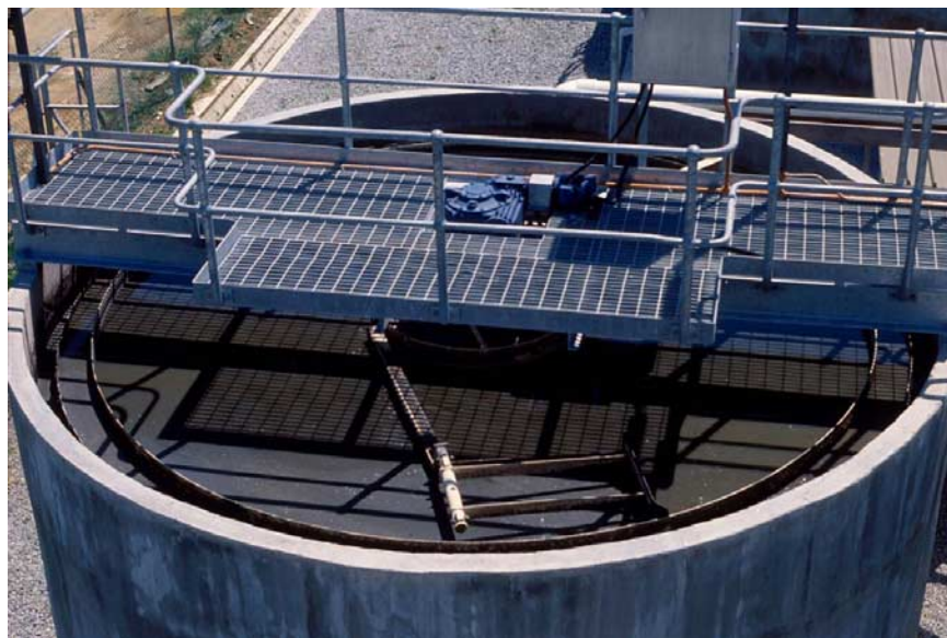
Fig. 6.2.1. Gravity thickener at a large pig farm's wastewater treatment plant.
