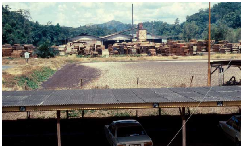
Fig. 10.3.1. Anaerobic lagoon for POME treatment. The dark brown scum layer which appears almost “crusty” is useful for excluding air from the anaerobic process occurring beneath it.
