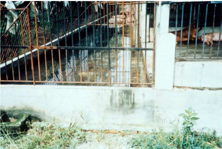
Fig. 8.1.2. Pig pen at a small farm. These pens are usually manually flushed by the farmer. The drain conveying the wastewater to the treatment plant may be seen on the LHS of the picture. This drain also serves to drain rainwater running off the roof which is undesirable as it unnecessarily increases the hydraulic load on the treatment plant during rain storms.
