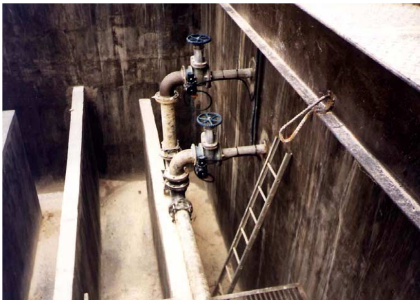
Fig. 3.7.1. Labyrinthine-type disinfection tank at a STP. The tank has been drawn down for maintenance. The arrangement of the baffles generates eddies which help in the mixing.
