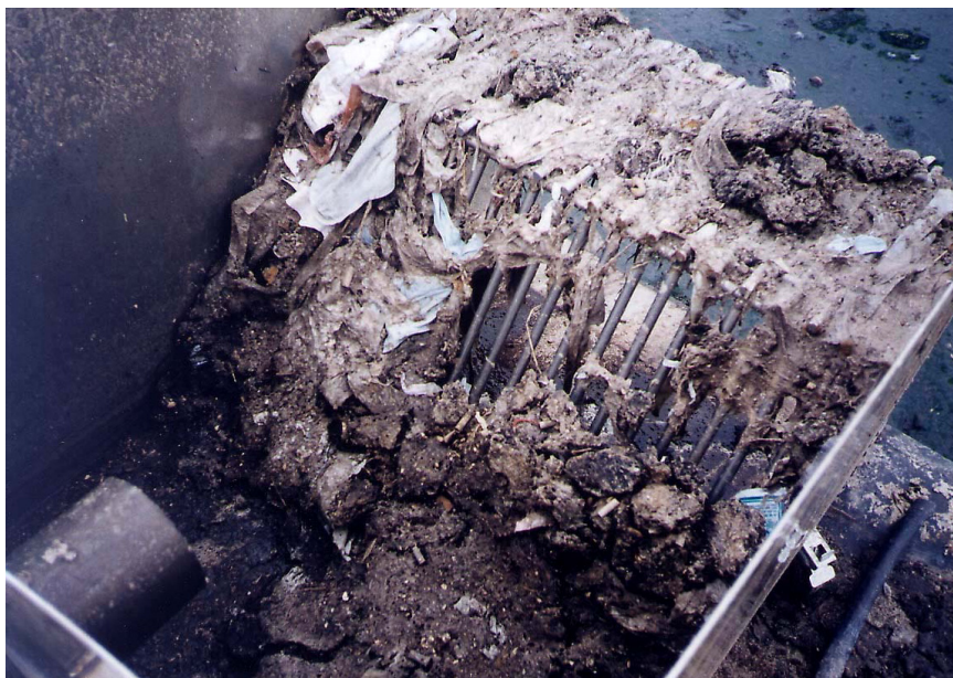
Fig. 3.2.1. Example of screenings collected on a manually cleaned rack. Note the gross material which includes pieces of paper and plastic wrapping. These can blind the screen unless regularly removed.
