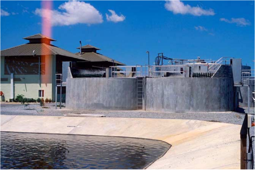
Fig. 8.3.2. Oxidation ditch system for (anaerobically) pretreated piggery wastewater. This is a pair of oxidation ditches fitted with rotor brushes for aeration.
