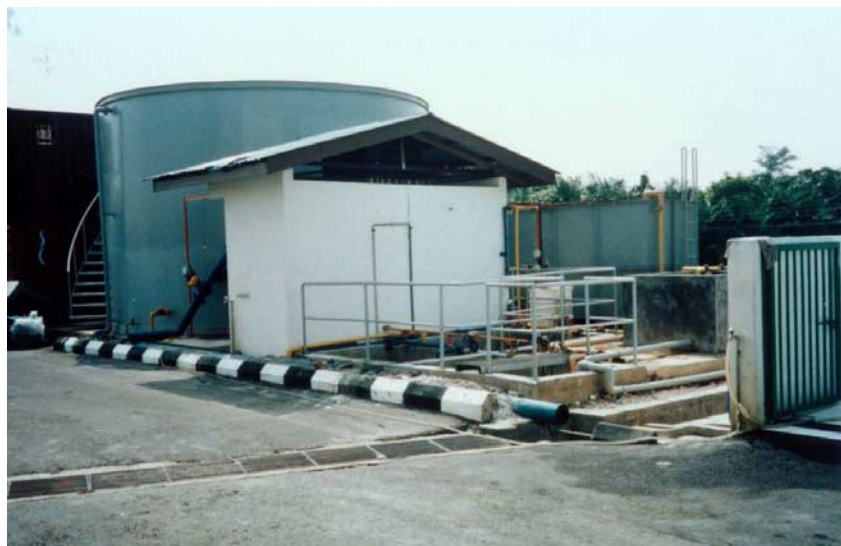
Fig. 7.3.1. Single reactor aerobic SBR for personal care products manufacturing wastewater treatment.
