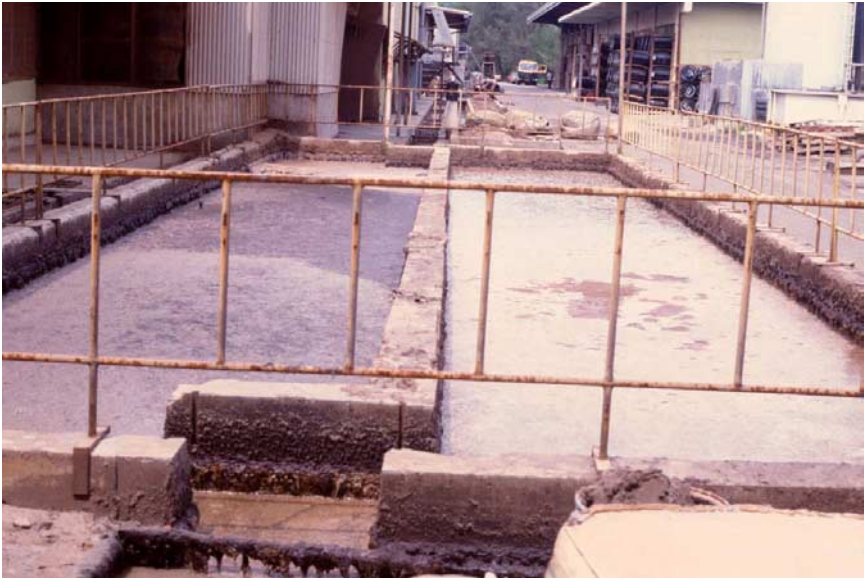
Fig. 4.3.1. Two-chambered aerated equalization tank at a lanolin extraction IWTP. The RHS chamber was being aerated while the LHS chamber was not at the time this picture was taken. The mixture of O&G and fine particulates make fouling of the equalization tank a recurring and serious maintenance issue. The material on the walls and pipe (foreground of the picture) gives an indication of the fouling. The latter had to be removed regularly to reduce the incidence of odours and slippery work surfaces.
