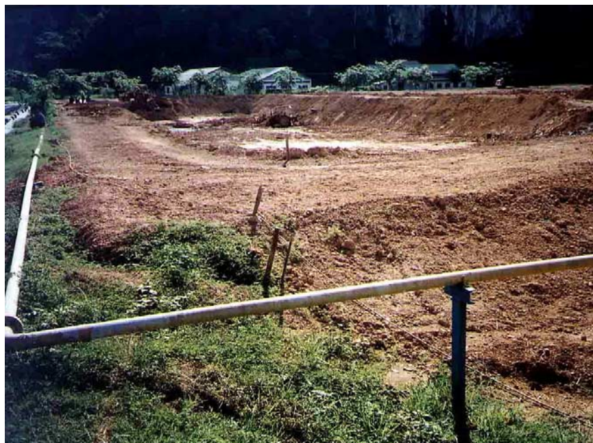
Fig. 5.5.1. Two anaerobic lagoon cells under construction. Note that the lagoon cells had not been lined nor had the bunds been fully constructed. The reinforced concrete inlet and outlet works had yet to be constructed.
