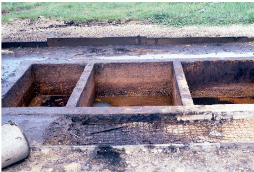
Fig. 4.2.4. The baffled tank O&G trap at a palm oil refinery provides for more quiescent conditions to allow for greater removal of O&G than what is possible with the simple trap shown in Fig. 4.2.3. In traps of this type, the O&G accumulated on the wastewater surface in each chamber is manually removed at intervals.
