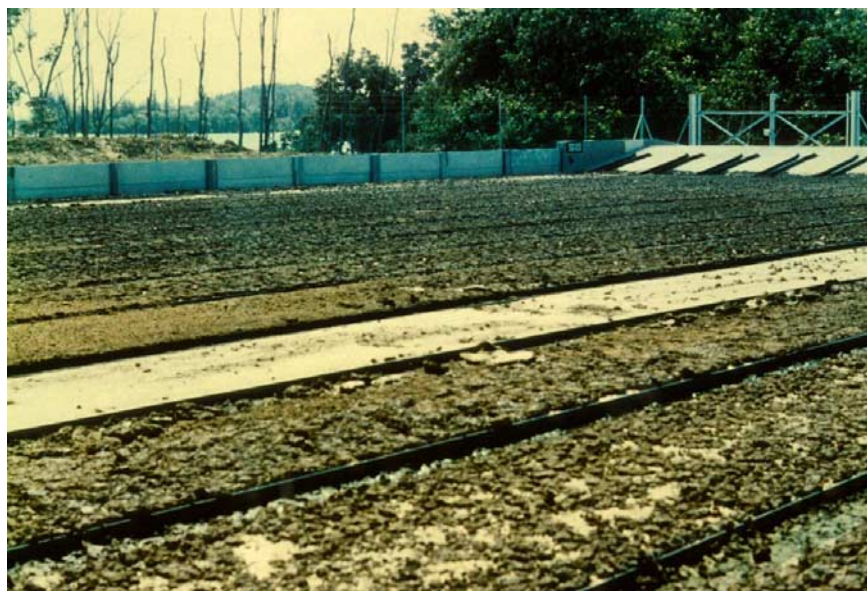
Fig. 6.5.3. Large drying beds fitted with running tracks for mechanical cake removal. These beds serve an industrial scale piggery farm.
