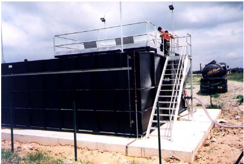
Fig. 3.8.2. Package STP based on the SBR for a small community of 2000ep. Note the steel plate construction of the vessels. These can be welded together relatively quickly and mounted on the concrete plinth.
