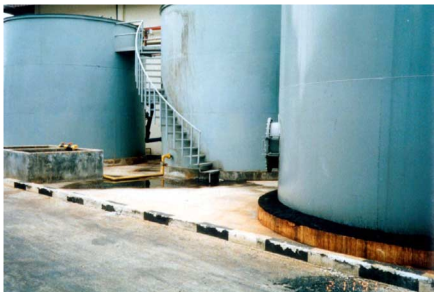
Fig. 10.3.4. Twin-tank aerobic SBR for PORE treatment. The third vessel on the LHS is a treated wastewater storage tank. Treated effluent quality from the SBRs had been found adequate at this refinery for use in its cooling towers. The rectangular structure in the foreground on the left hand side is a pair of sludge drying beds. Treatment of physical refining wastewater does not generate large quantities of sludges. This is unlike chemical refining wastewater which requires coagulant assisted dissolved air flotation before biological treatment. The use of coagulants results in much larger quantities of sludge requiring disposal.
