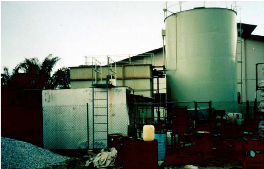
Fig. 5.5.4. IWTP comprising of a SBR and anaerobic filter (RHS cylindrical reactor) for fructose wastewater.
