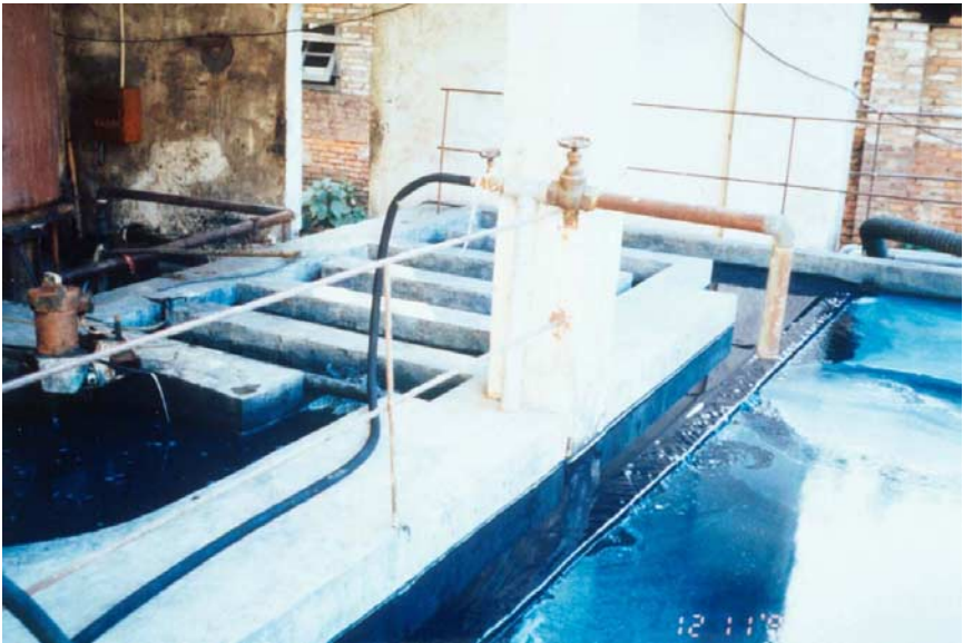
Fig. 4.4.3. Labyrinthine-type flocculator (LHS) at a IWTP for a textile dyehouse. Dosing of the flocculant from a pipe just before the start of the first baffle of the flocculator can be seen on the LHS of the picture.
