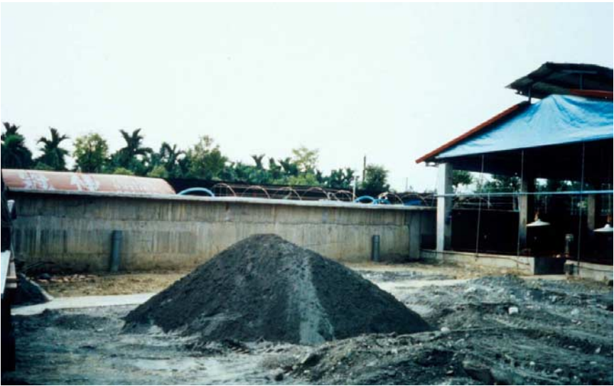
Fig. 8.3.3. A cyclic piggery wastewater biotreatment system. The anaerobic SBR (LHS — With the red-mud membrane cover) is followed by the aerobic SBR (RHS — Without the cover).
