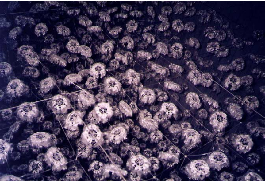
Fig. 5.4.3. “Fibrous” support medium mounted within an anaerobic filter (view from the top).
