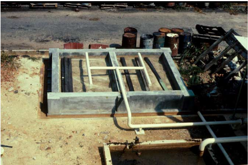
Fig. 6.5.2. A pair of newly constructed sludge drying beds showing the gravel bed, underdrain, and sludge application pipes above.
