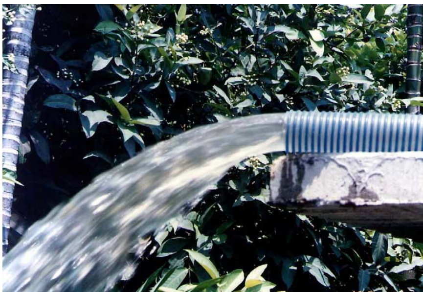
Fig. 8.4.3. Relatively color-free treated piggery wastewater. This followed reformulation of the animal feed.
