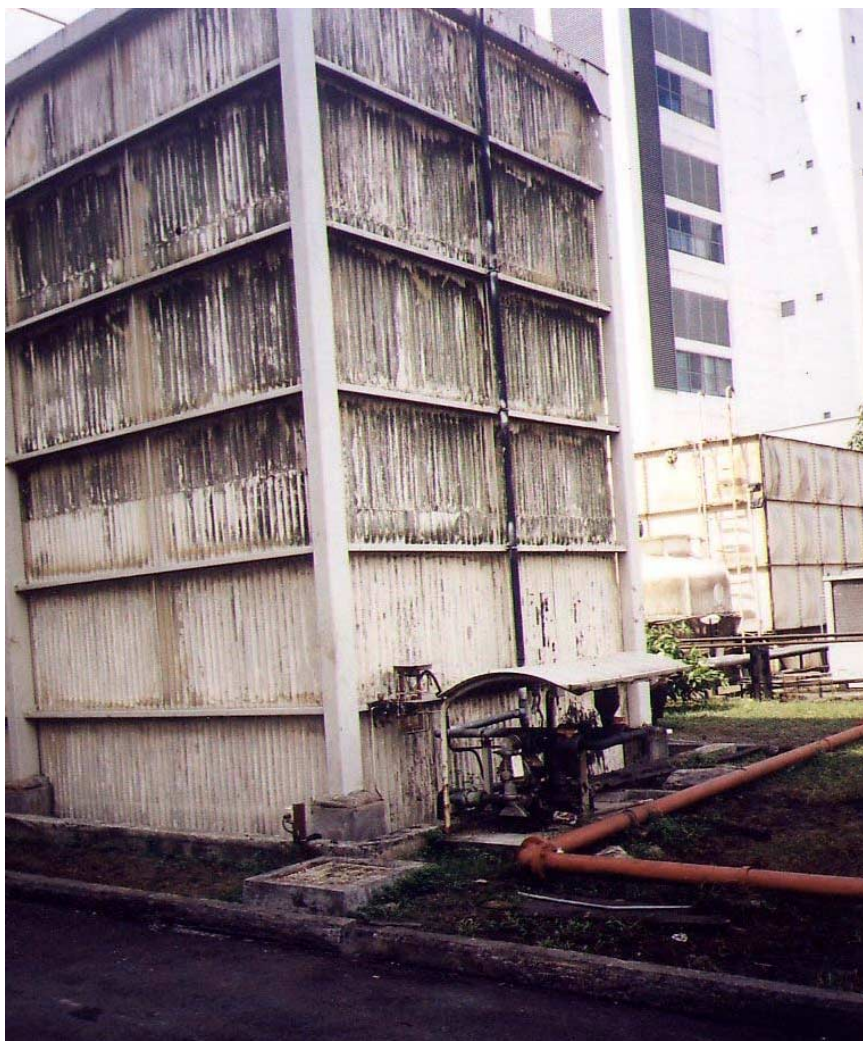
Fig. 5.4.2. Roughing trickling filter with forced ventilation at a coffee extraction plant.
