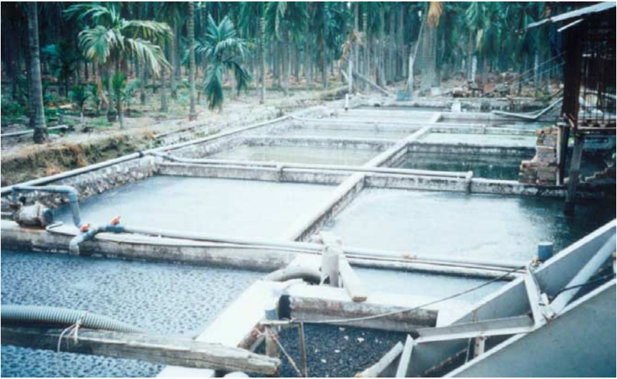
Fig. 8.3.1. Anaerobic ponds (which have been staged) for piggery wastewater treatment.
