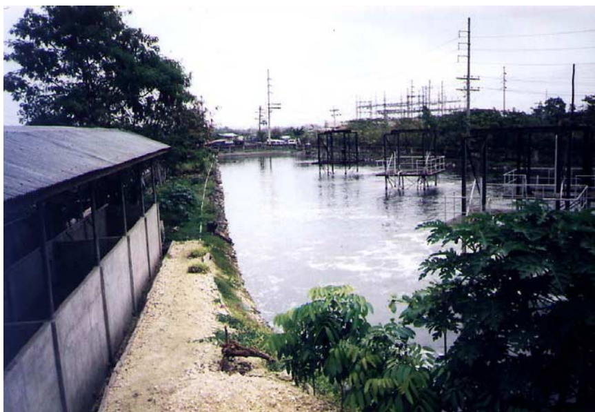
Fig. 9.3.3. An aerated lagoon at a slaughterhouse. The three sets of piers are for mounting surface aerators. The animal holding pens are on the left hand side of the picture.
