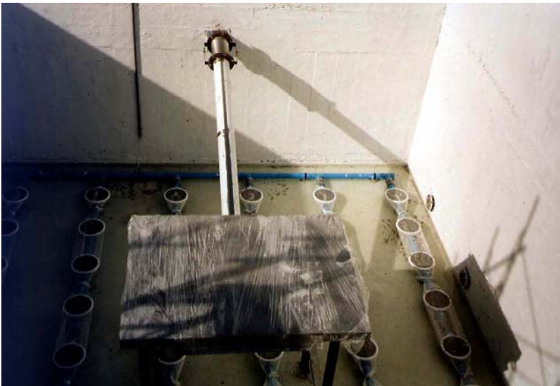
Fig. 3.6.4. Decanter assembly in a cyclic reactor (SBR) with the overflow weir in the decanter head (foreground) (decanter and diffusers installed but still to be commissioned). The decanter assembly is articulated at the point where the decanter head meets the decanter arm and where the arm meets the discharge pipe exiting the reactor's wall.
