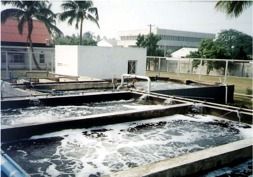
Fig. 3.4.1. Activated sludge plant for sewage treatment where the bioprocess is a combination of suspended and attached growth. The submerged biofilm support modules are located along a line running longitudinally and down the center of the tank.
