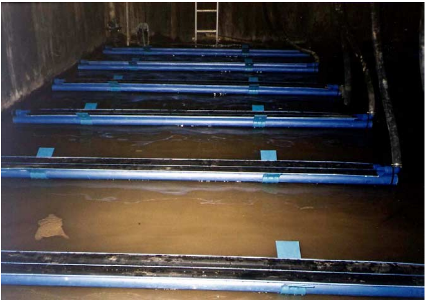
Fig. 5.6.2. Tubular diffusers installed on the bottom of an aeration vessel.
