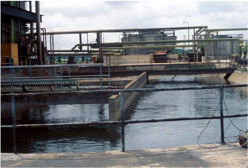
Fig. 5.6.1. An oxidation ditch at a palm oil refinery. Note the central wall which divided the basin into two halves and thereby forming the “race track” configuration.
