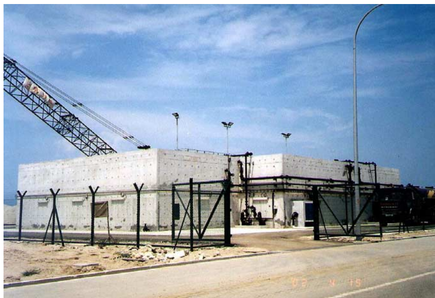
Fig. 3.8.3. Mid-sized STP based on the SBR for 20000ep. This larger STP, compared to the example shown in Fig. 3.8.2, has been constructed using reinforced concrete. The decision between using steel or concrete is often based on the speed of construction required and the cost of the construction materials.
