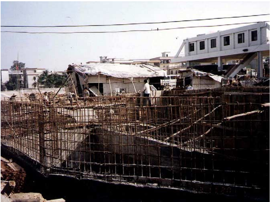
Fig. 5.3.1. The “trapezoidal” tank under construction in the foreground was to be a SBR vessel. The SBR was selected because it is least sensitive to vessel configuration. Available space at the site did not permit construction of vessels with “regular” shapes and still achieve the required hydraulic capacity.
