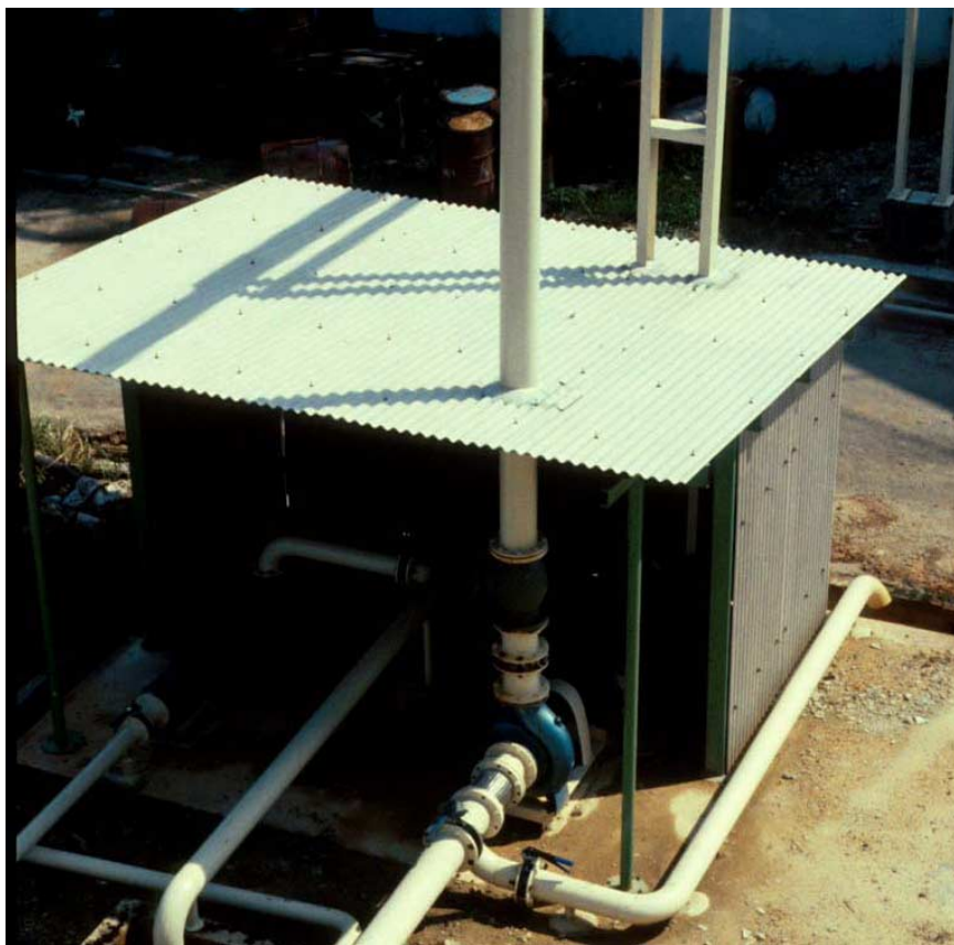
Fig. 10.3.3. pH correction station at a PORE treatment plant. This is a single stage pH correction station with sodium hydroxide.
