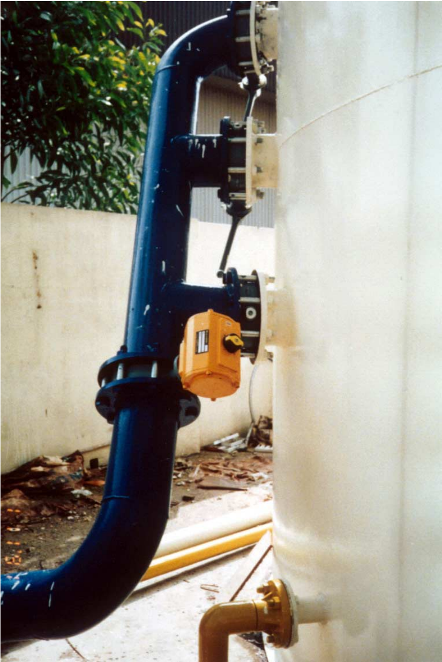
Fig. 5.6.4. Multiple fixed point decanter on a SBR which allows selection of any one of three preset decanted levels. The lowest and smaller pipe is for desludging.
