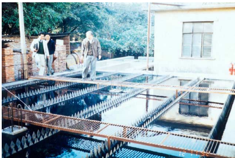
Fig. 4.4.4. Rectangular clarifiers following coagulation/flocculation at a textile dyehouse. Rectangular vessels may be easier to arrange in a more space-saving manner compared to circular vessels.
