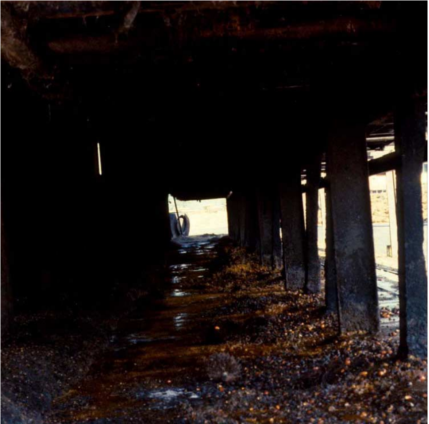
Fig. 10.1.1. Palm oil FFB receiving bay. The pressure of piled up fruit bunches as these are unloaded onto the loading bay above resulted in some oil being squeezed out and this dripped onto the ground shown on this picture. This oil is collected by surface drains and at least a portion of it would make its way to the wastewater treatment plant.
