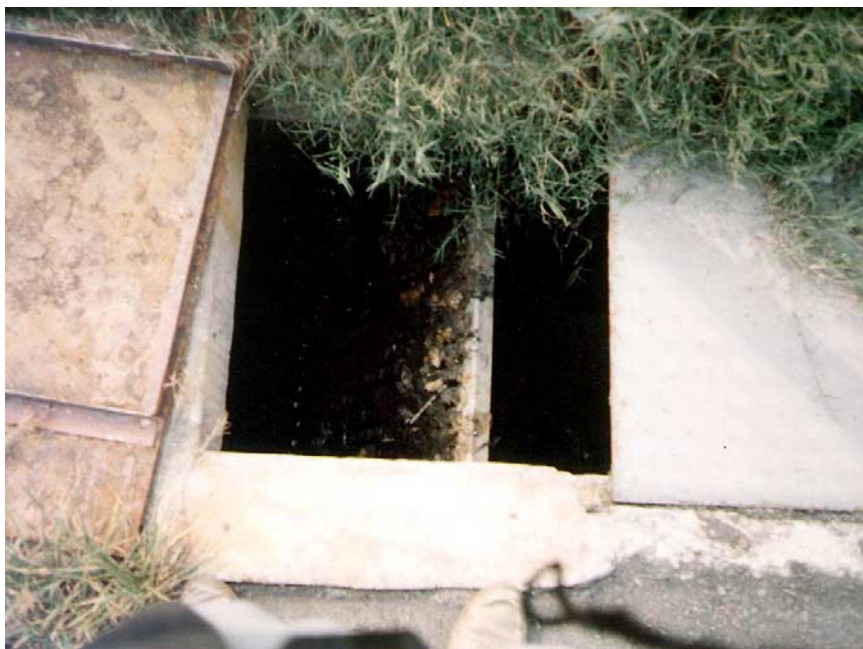
Fig. 4.2.2. Covered drain leading to the collection sump of an IWTP. The (removed) cover had been placed over a coarse screen. The easily removable covers facilitate the removal of screenings from the screen. The drain is shallow because the distance between the factory and IWTP is small.
