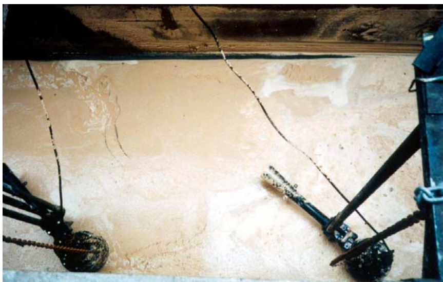
Fig. 5.6.3. Jet aerators in a reactor at an IWTP for a milk canning factory. These are normally submerged and are shown exposed in the picture because the reactor has been drawn down for maintenance.
