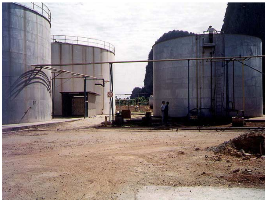
Fig. 5.5.2. A cluster of three anaerobic digesters used at a sugar mill. Such digesters can also be found at palm oil mills.
