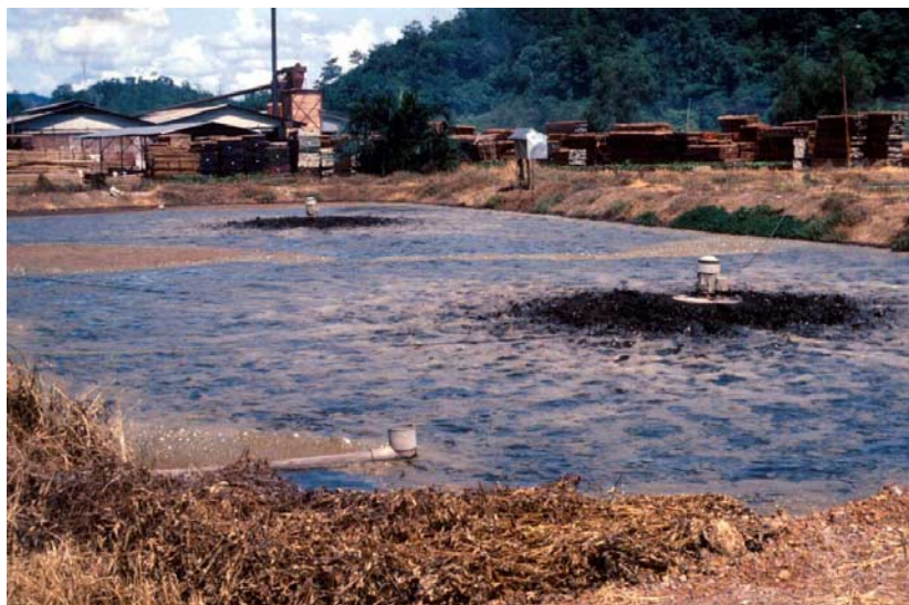
Fig. 10.3.2. Aerated lagoon treating POME. Typically such rectangular-shaped lagoons are designed to be aerated with at least 2 surface aerators for better mixing of the lagoon's liquor.
