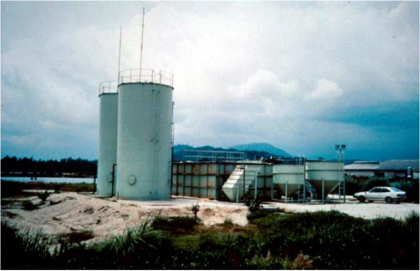
Fig. 5.5.5. IWTP with hybrid anaerobic reactors (the pair of cylindrical reactors on the LHS) and activated sludge process for rubber thread wastewater.
