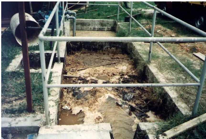
Fig. 9.3.2. Wastewater collection sump at a poultry slaughterhouse. The scum comprised feathers, O&G, and blood.
