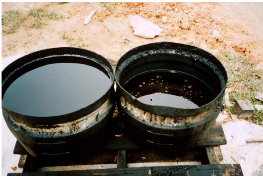
Fig. 4.2.5. Lubricating oil collected from the O&G trap at a soft drinks bottling plant. The lubricating oil came from excess oil applied to the bottle conveyor belt system. This dripped onto the floor and was eventually washed into the collecting drains leading to the IWTP.
