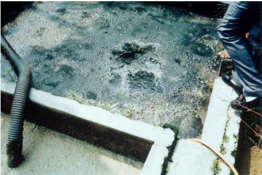
Fig. 8.2.1. Piggery wastewater collection sump. The “frothy” appearance on the surface of the wastewater was caused by the release of gases arising from fermentation. A large component of the organic pollutants in piggery wastewater is easily biodegradable.
