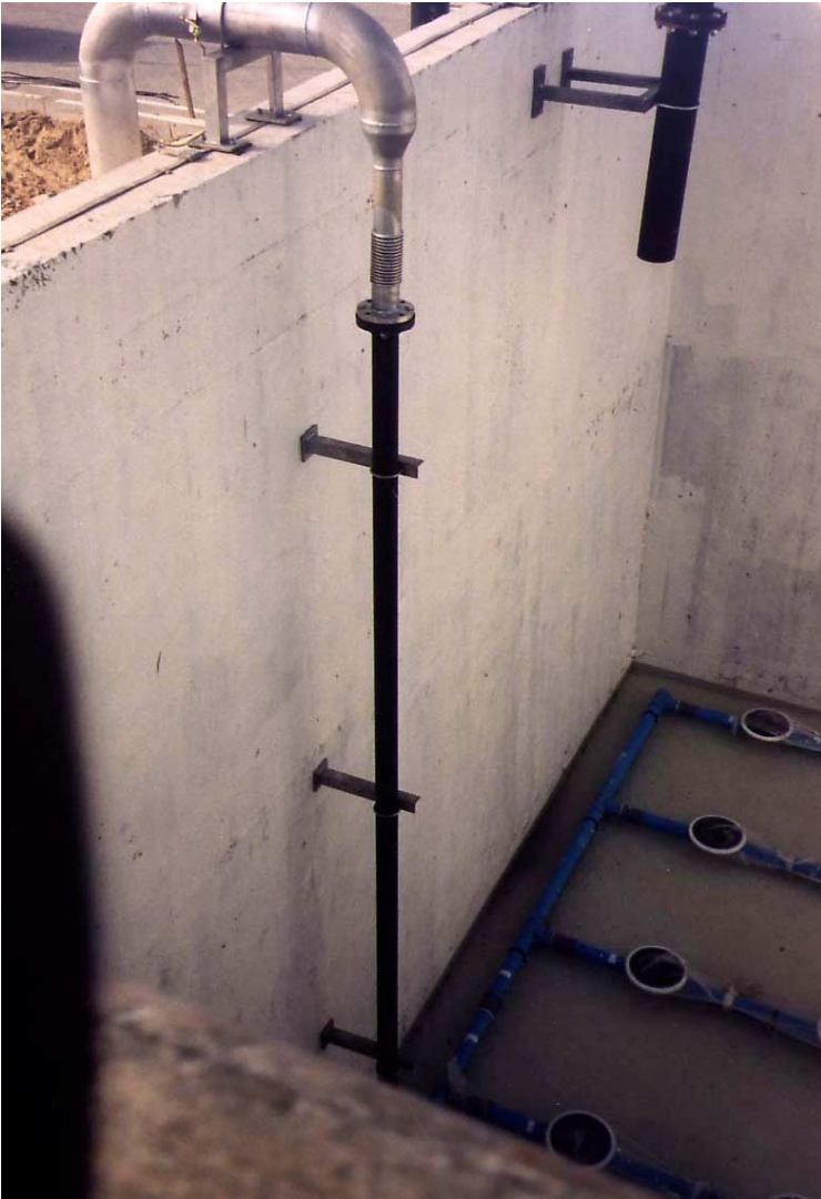
Fig. 3.6.2. Air header and circular membrane diffusers in a reactor drawn down for maintenance.
