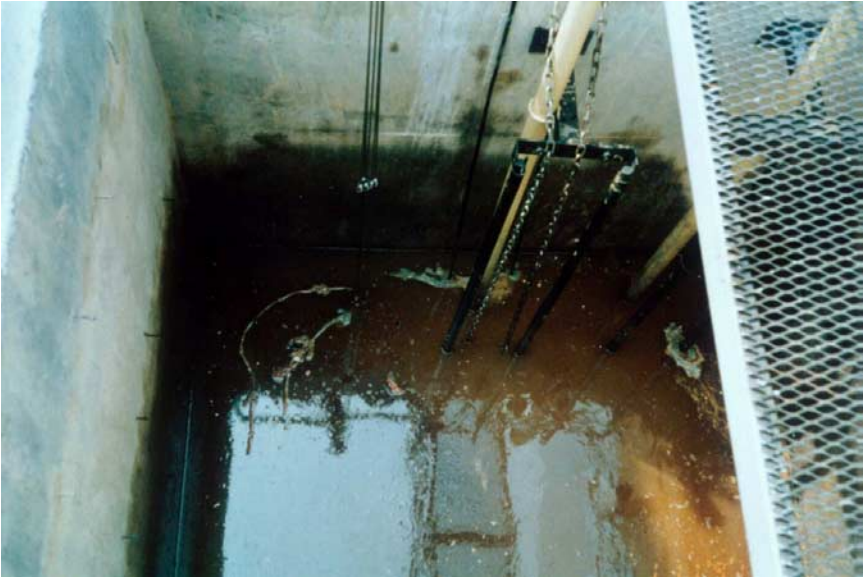
Fig. 4.2.1. Shallow wastewater collection sump at a personal care products factory. Submersible are located in this sump to lift the wastewater to the next unit process in the IWTP. The sheen on the water surface suggests the presence of O&G.
