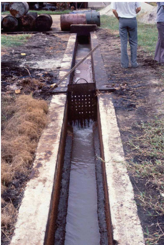
Fig. 4.2.3. Baffle plate O&G trap inserted into a surface drain leading to the IWTP at a palm oil refinery. The effectiveness of such a simple device may be seen from the O&G accumulated behind the baffle plate. While not reducing the wastewater's O&G content to the required levels, the trap significantly reduced the O&G load which would otherwise be imposed on the next unit process.
