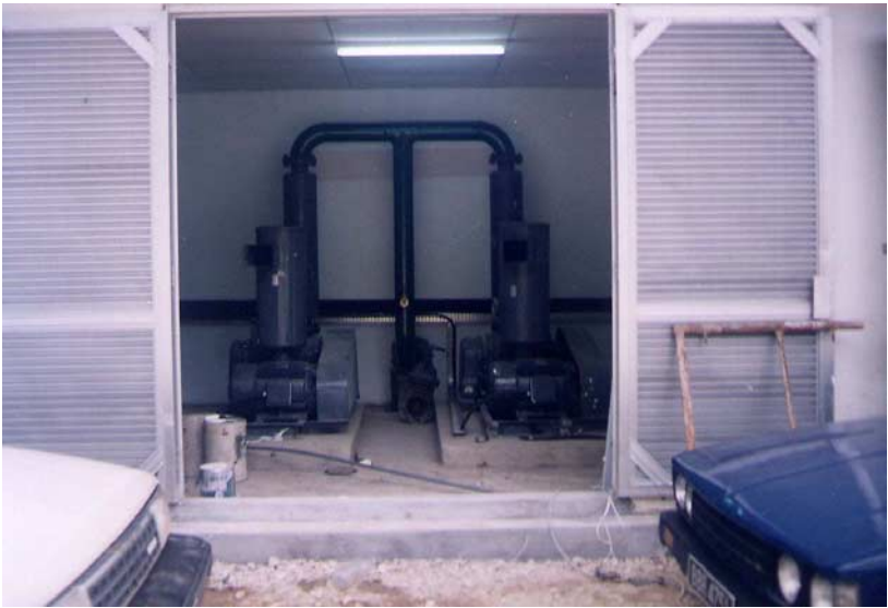
Fig. 3.6.3. Blowers sited in a blowerhouse which also served to attenuate noise (blowers installed but still to be commissioned).
