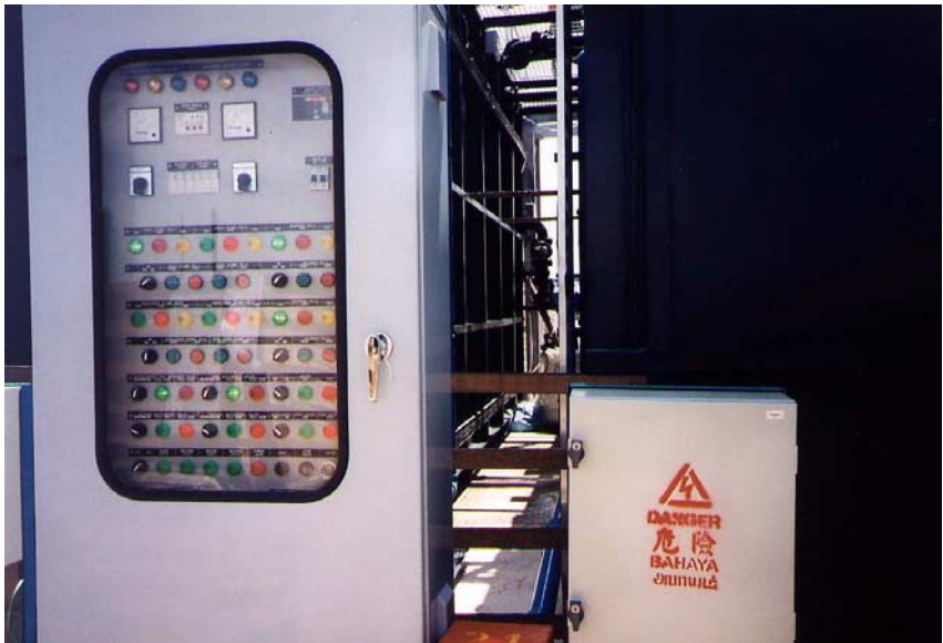
Fig. 3.8.1. Central control panel at a small STP.
