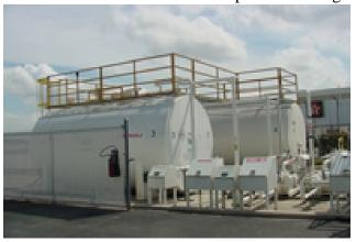
Figure 17 - Horizontal tank.
