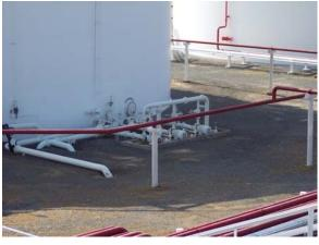
Figure 8 – Red piping showing foam piped to sub-surface foam system.
