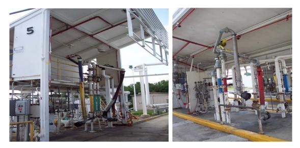
Figure 3 – Typical loading racks found in the NOVA region.
