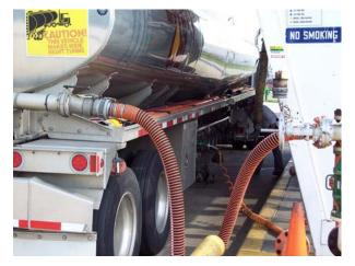
Figure 4 – Loading rack with vapor recovery, electrical ground, and fuel fill hose attached.
