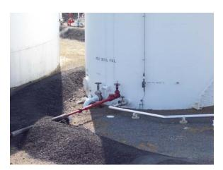
Valves, connections, and couplings are also located within the dike area and serve to terminate the flow of petroleum product from the bulk storage tank to a loading rack or transmission pipeline.
