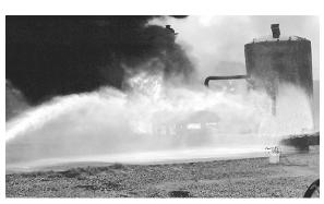
Figure E3: Rain-down method of foam application. Reprinted from Essentials of Fire Fighting, 4<sup>th</sup> ed, IFSTA
