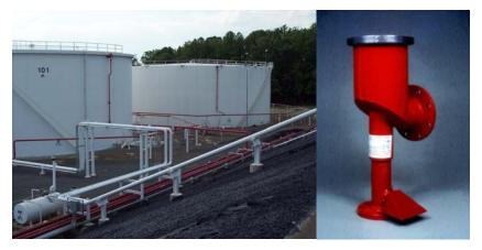
Figure 10 – Fixed and semi-fixed foam protection systems designated by red piping. The figure on the right is a type II foam chamber.
