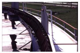
Figure 13 – Floating roof seal.
