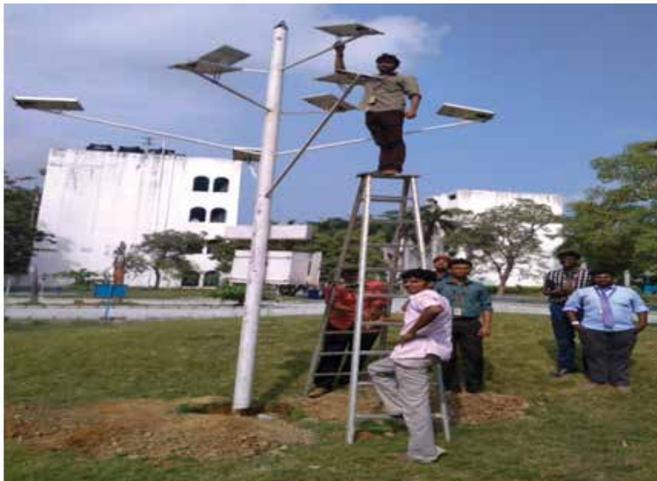
Solar tree top view
