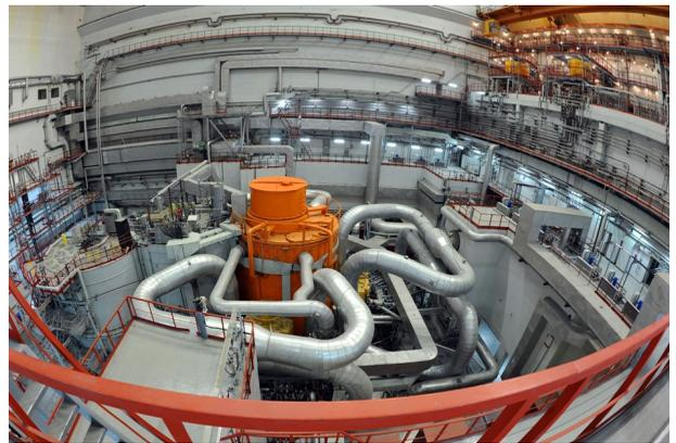
The sodium cooled fast reactor Beloyarsk 4 entered commercial operation 31 October 2016. Even though it does not fulfil all of the Generation IV criteria, it demonstrates that technology for large breeder reactors is in place. Photo credit Rosatom
