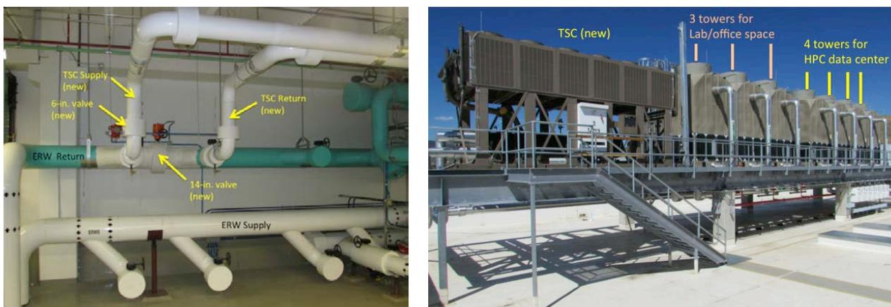
**Figure 3** (a) Pipe modification to the ERW loop and (b) TSC installation.
