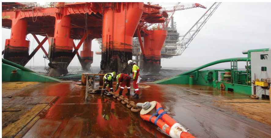
Viking SeaTech workers inspect a mooring assembly for an offshore platform
