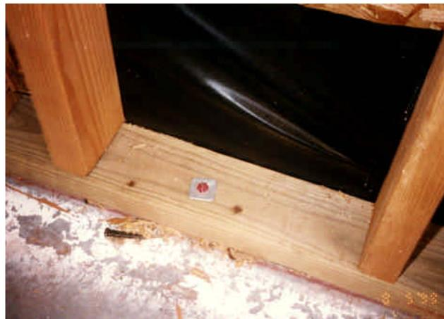
Figure A2.2. Attachment of bottom plate by shotpins. [Photograph © T. Marshall, used by permission]
