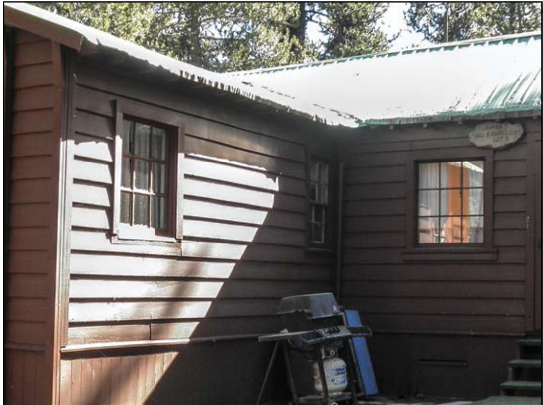
Figure 5—Part of the windowsill broke off of this recreation residence's left window. Replacing it with a windowsill that exactly matches the other windows is routine maintenance.
