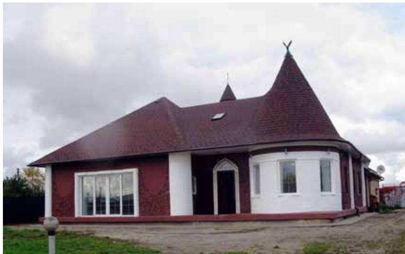
**Figure 40.** The first residential building in Europe printed with a 3D construction printer. Yaroslavl (Russia). Source: AMT-SPETSAVIA Group (Russia) – [www.specavia.pro](http://www.specavia.pro), CC BY-SA 4.0, <https://commons.wikimedia.org/w/index.php?curid=74334750>.
