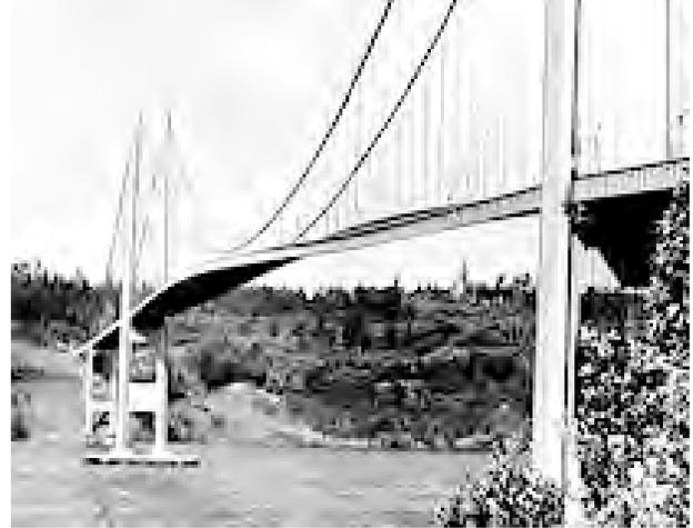
Vortices around its deck caused by winds of 35 – 40 mph caused the bridge to begin rising and falling up to 5 feet, forcing the bridge to be closed at about 10 am. The amplitude of motion eventually reached 28 feet.
