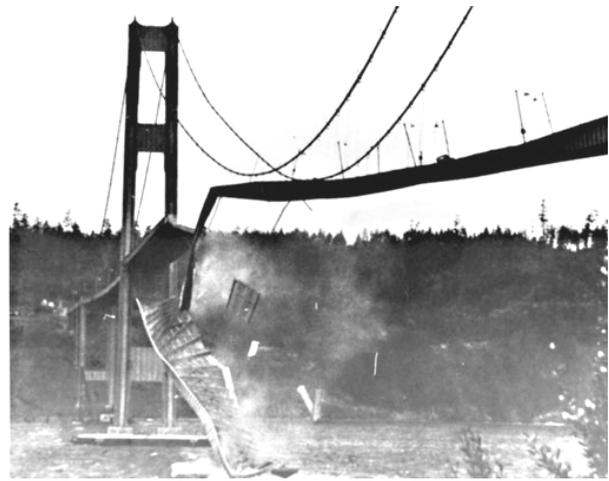
At 10:30 am the oscillations had finally caused the center span floor panel to fall from the bridge. The rest of the breakup occurred over the next 40 minutes.
