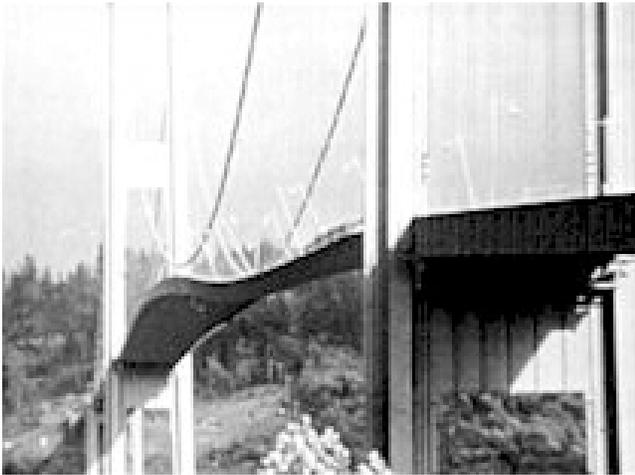
The Tacoma Narrows Bridge on November 7, 1940. Workers on the construction of the bridge had referred to it as “Galloping Gertie” because of the unusual oscillations that were often present. Note nodes at the towers and in the center of the deck. This is the second mode.
