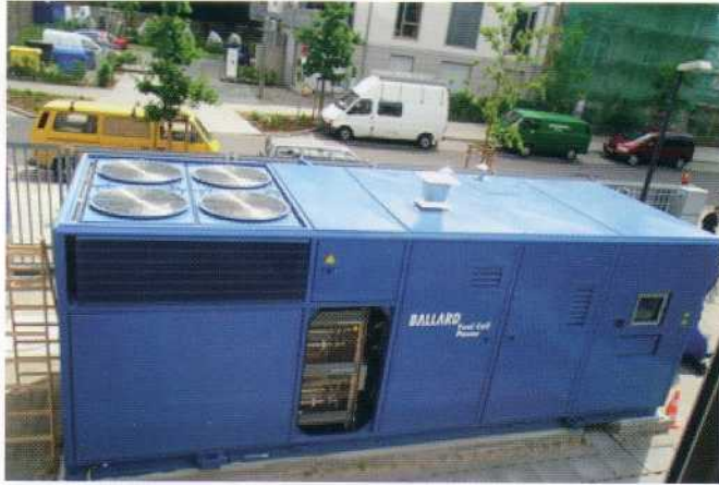
CHAPTER 8, COLOR FIGURE 8.7 The 250-kW Ballard Generation Systems PEMFC power plant installed in Berlin in 2000. (Photograph courtesy of Ballard Power Systems.)
