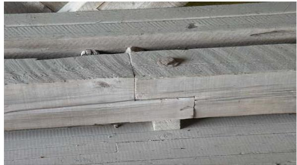
**Figure 6.6—Gap under guardrail allows debris to be washed away. Compare with guardrail in Figure 6.2 that rests directly on the wearing surface (Willard Covered Bridge, 1871, Windsor County, Vermont).**
