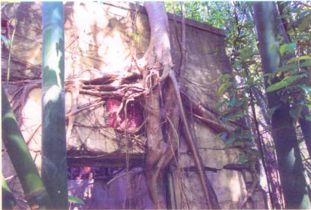
Photograph 3: DETAIL OF PARTIAL SOUTH ELEVATION SHOWING TREE GROWING FROM WALL WITH ROOTS EXTENDING TO SIDES AND DOWN.
