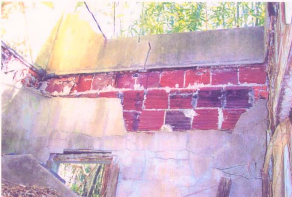
Photograph 6: DETAIL OF COLLAPSED ROOF OF LAUNDRY ROOM SHOWING PARAPET ABOVE ROOF, FLASHING DETAILS, ROOF RAFTER LINE AND ADJACENT STUCCO.
