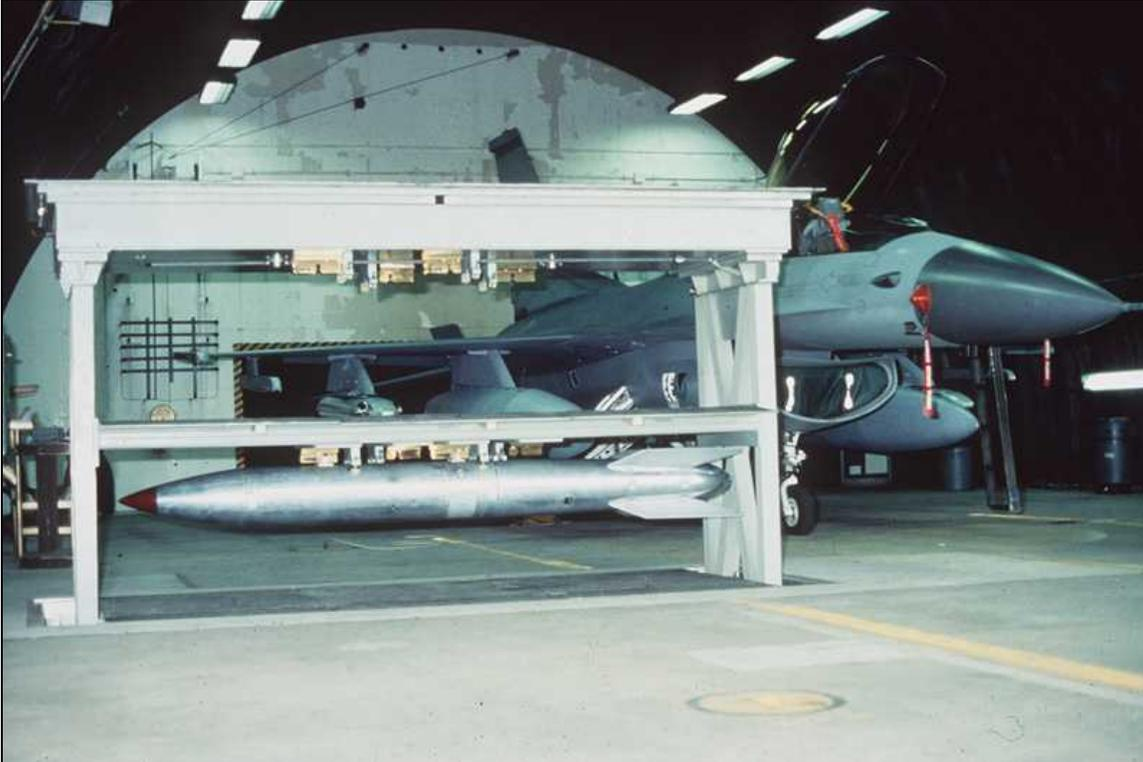
Elevated Weapons Storage Vault (WSV) with B61 body in Protective Aircraft Hangar with F-16 in the background. Notice the offset twin hangars in the ceiling of the top rack enabling storage of two offset weapons on each level for a total of four weapons in the vault. *Source: U.S. Air Force.*
