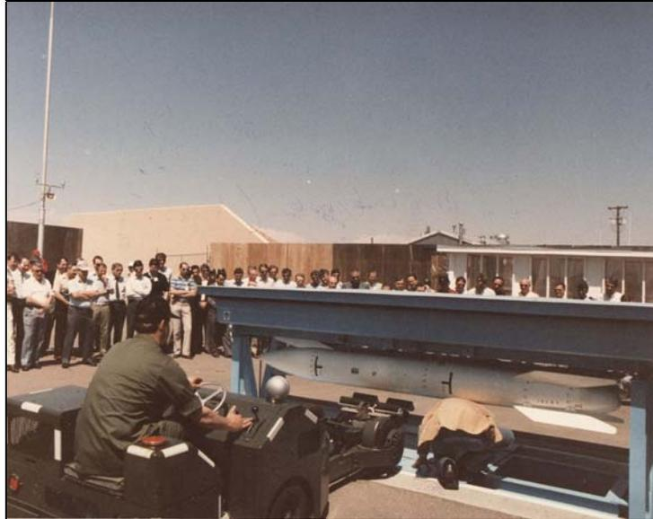
Loading demonstration of two B61 bomb shapes into the top bay of a Weapons Storage Vault (WSV) at Sandia National Laboratories. Notice the tailfins of the two bombs hanging in opposite directions, enabling storage of two weapons in each bay.
