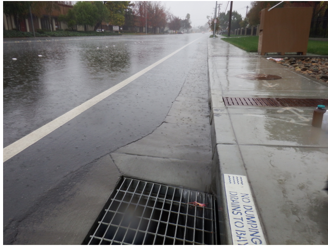
Figure 8. Stormwater bypassing the TWF inlets and flowing directly into the storm drain untreated was observed during storm events with rainfall intensities of 0.33 in/hr and greater.
