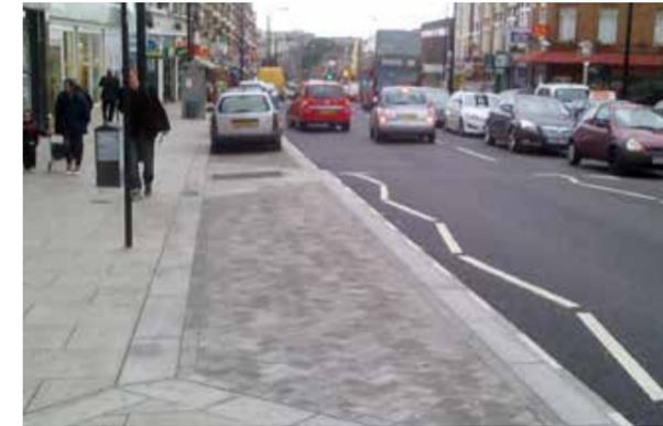
Footway level parking and loading pads act as an extension to the footway. Changes in materials should be considered when using this type of treatment so that blind and partially sighted people can clearly differentiate between pads and the footway
