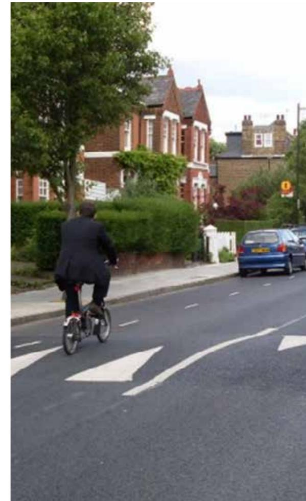
Sinusoidal humps used in London
